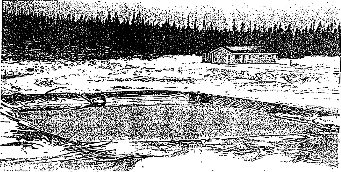
6(a) Reagent Containment Pond
