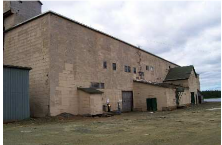
Photo 2: Main Mine Building.
