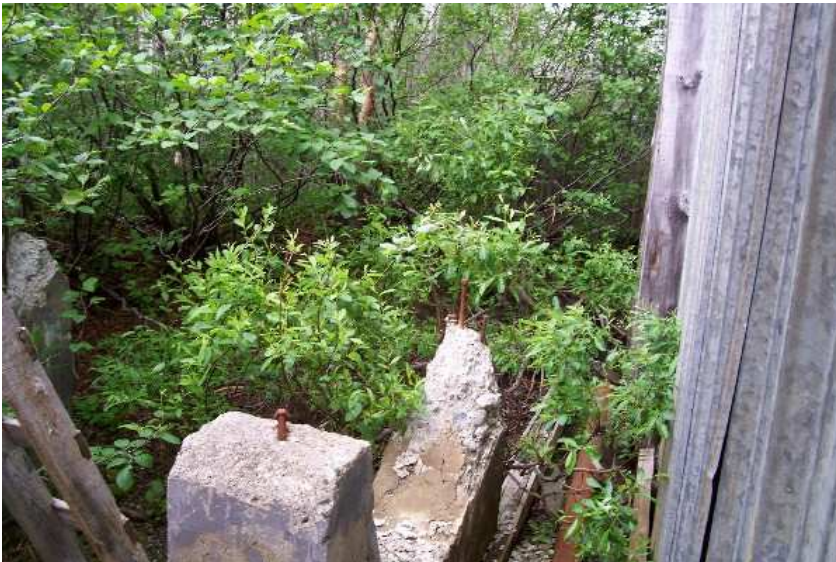
Photo 3: Former AST Cradle (1 of 2) behind Building No.2.
