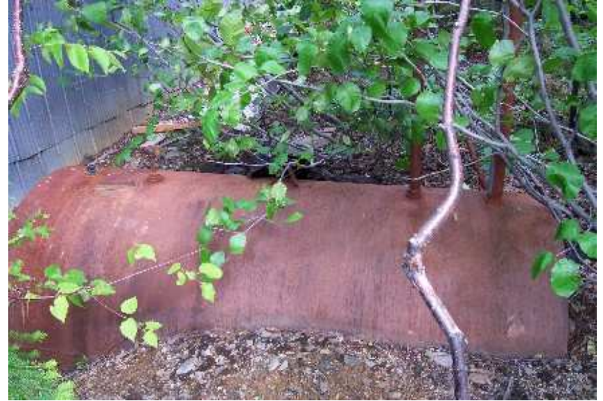
Photo 6: UST - Southwest Corner of Bunkhouse No. 2. (Bunkhouse Area)
