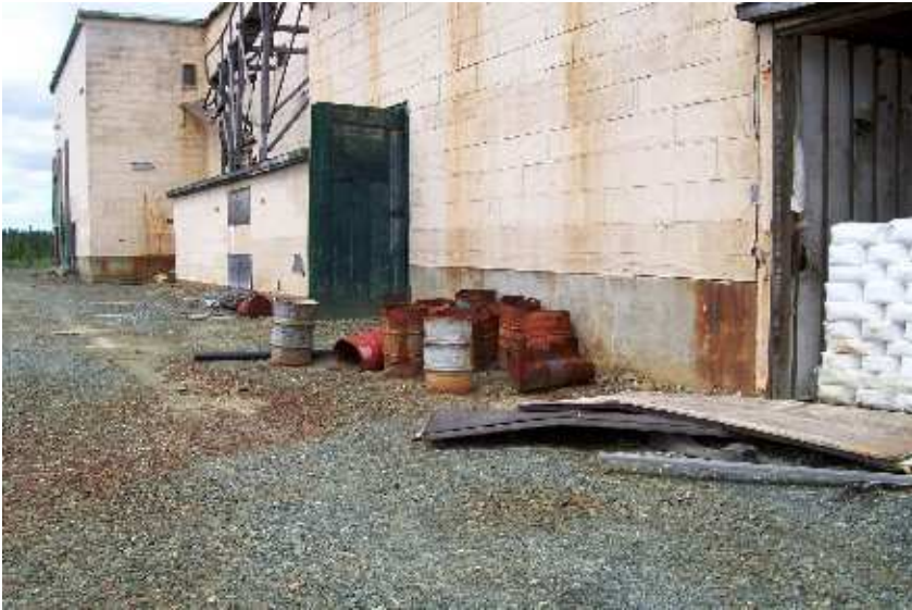
Photo 21: 45-Gallon Drums Filled with Sand and Gravel.
