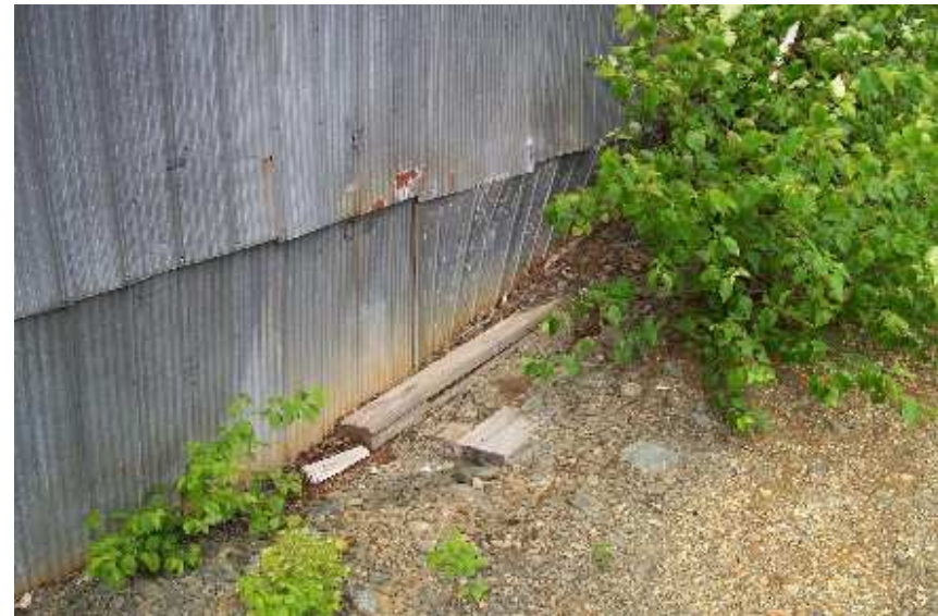
Photo 8: Potential AST Holding Pad on Southwest Corner of the Cookhouse.
