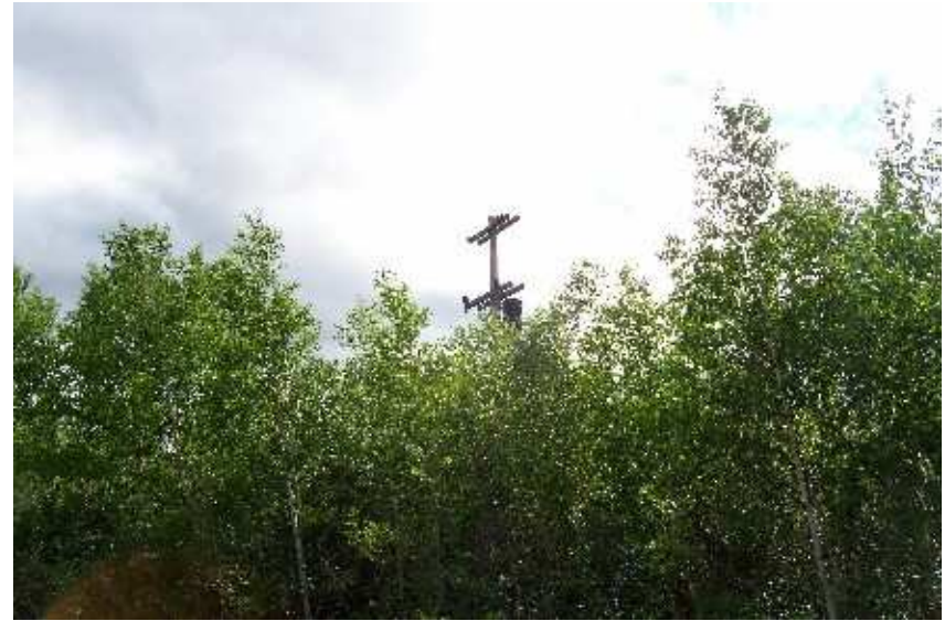
Photo 6: Transformer #2. (Northwest of Staff House)
