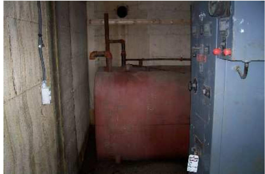
Photo 22: Main Mill Building - Two 200-Gallon ASTs.
