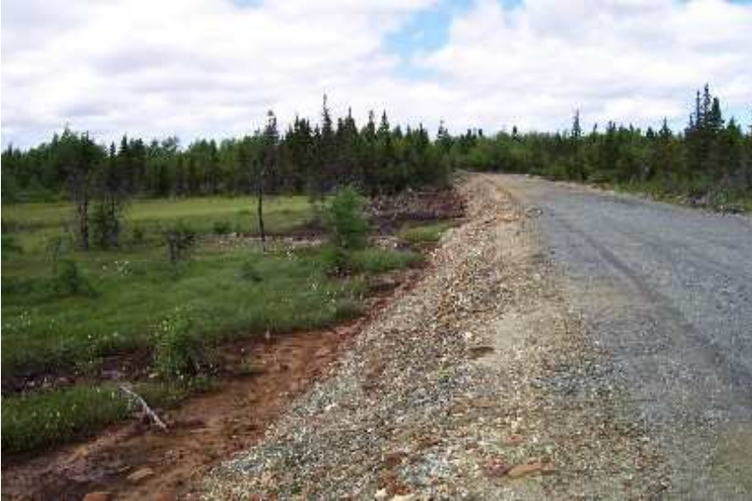
Photo 1: Main Access Road to the Rambler Mine. (Note the Potential Acid Generating Waste Rock and Stressed Vegetation)
