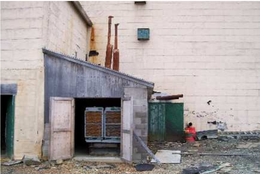
Photo 23: Main Mill Building - Generator.
