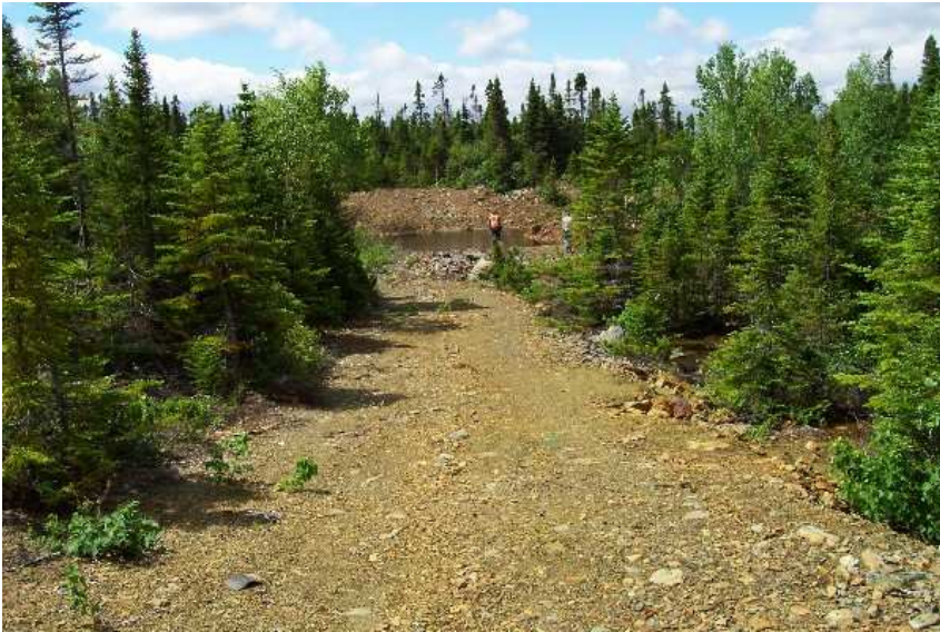
Photo 1: Access Road to Big Rambler Pond Mine. (Note the Potential Acid Generating Waste Rock)
