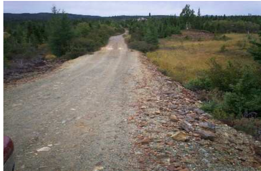
Photo 4: Alternate Access Road. (Note the Potential Acid Generating Waste Rock)
