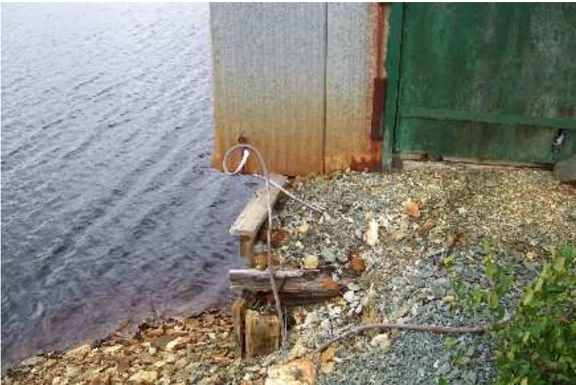
Photo 19: Pumphouse – Potential Fuel Lines.
