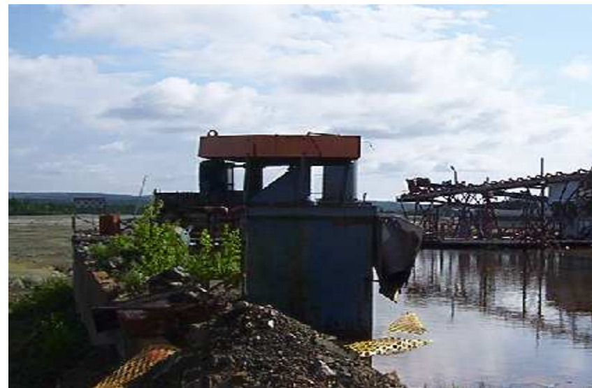
Photo 4: Metal Processing Equipment. (Note: Not a Fuel Storage AST)
