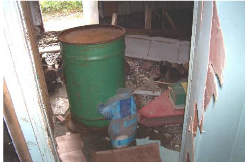
Photo 10: Drum - Sample Storage Area of Building No.2. (No Label - Empty)
