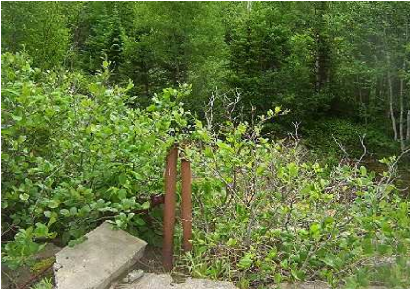
Photo 7: Possible Fill and Vent Pipe at Building No. 3. (Possible UST)
