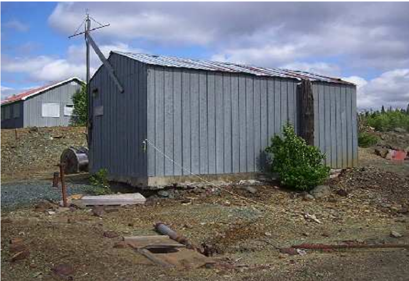
Photo 3: Gasoline UST and Diesel UST – Refueling Station. (Rambler Main Mine)
