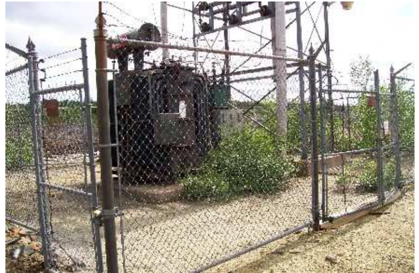
Photo 16: Pad-Mounted Transformer.
