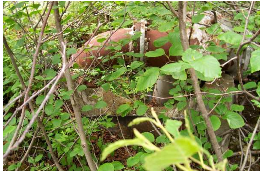
Photo 4: Former AST Cradle (2 of 2) behind Building No.2.
