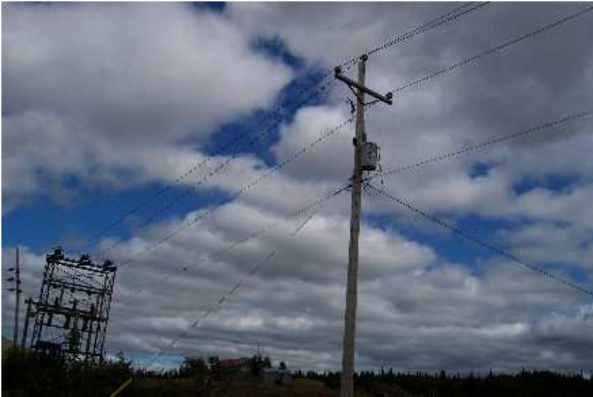
Photo 17: Pole-Mounted Transformer.
