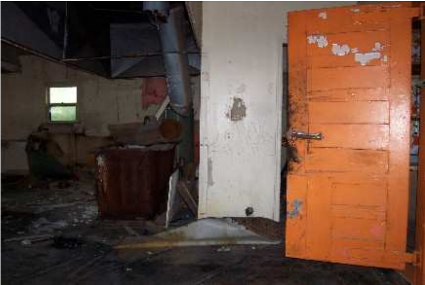
Photo 9: Oil Stove inside Cook House. (Note Hydrocarbon Odour Observed at this Location)
