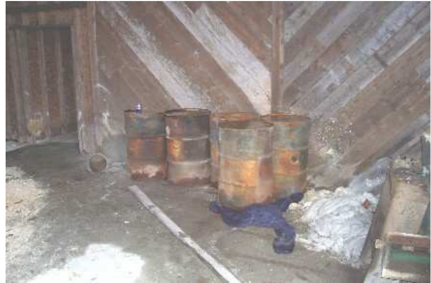
Photo 26: Full Drums inside Storage Shed. (Note the Discarded HazMat Suit)
