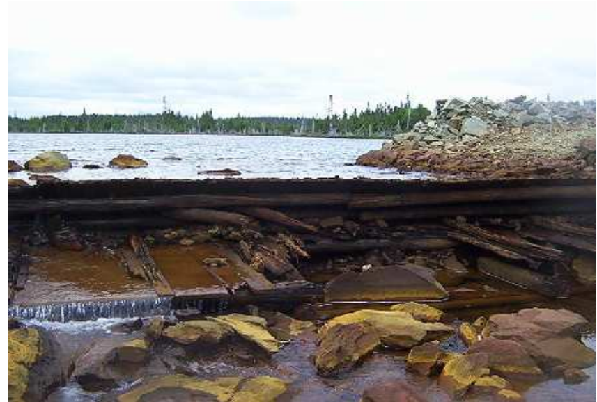
Photo 6: Wooden Spillway of Tailings Holding Pond.
