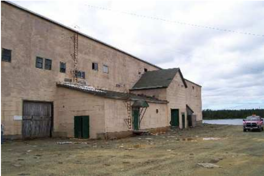
Photo 25: PCB Storage Area and Reagent Storage Area.
