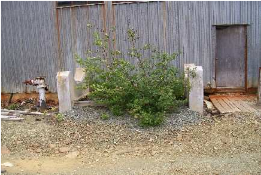
Photo 37: AST Cradle – Hoist Building.
