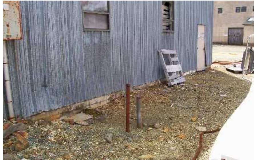
Photo 2: UST - Northside of Maintenance Garage. (Rambler Main Mine)
