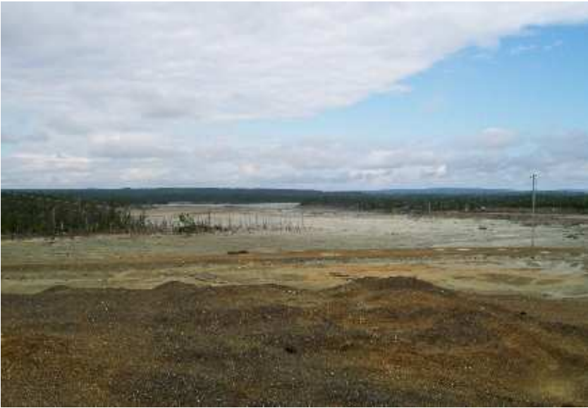
Photo 1: Overview of the Tailings Area. (Looking Northwest)
