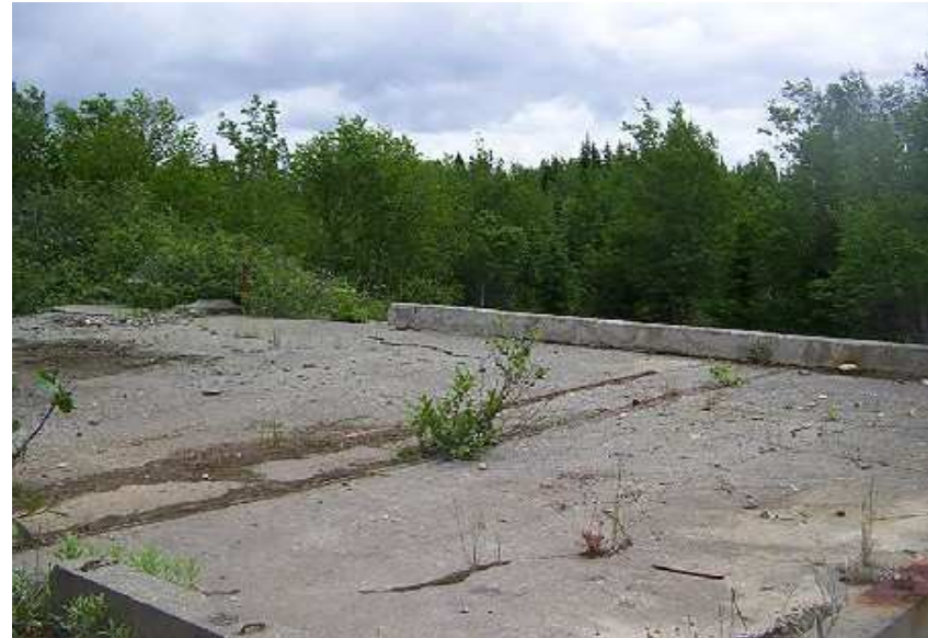
Photo 6: Concrete Foundation of Building No.3.
