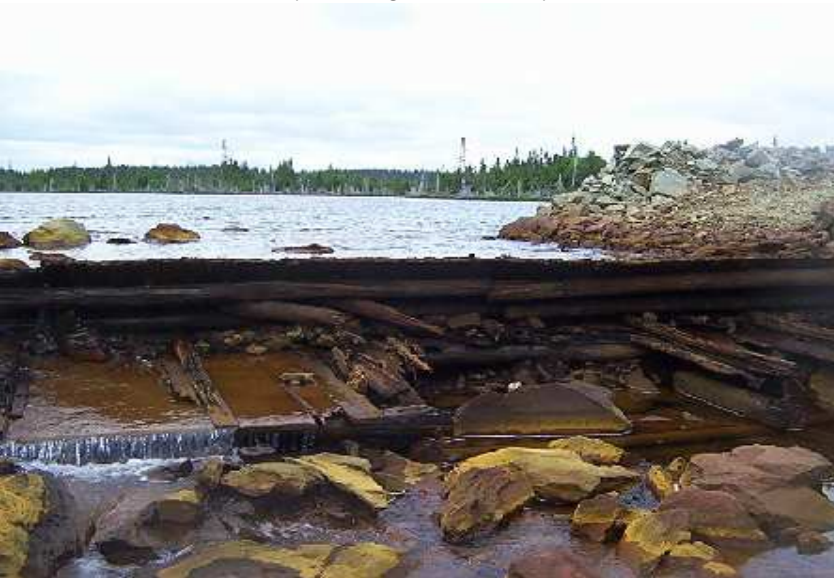
Photo 3: Wooden Spillway of Tailings Holding Pond.
