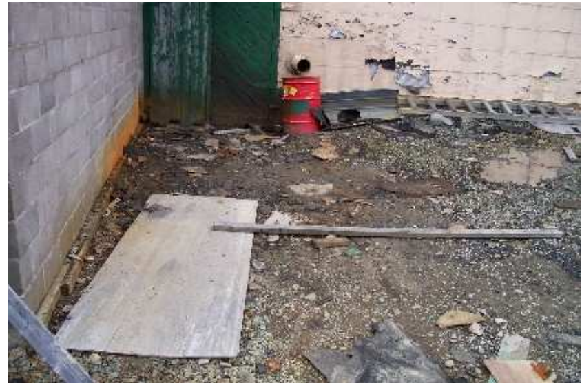
Photo 24: Stain Area – Downgradient of Generator and ASTs.
