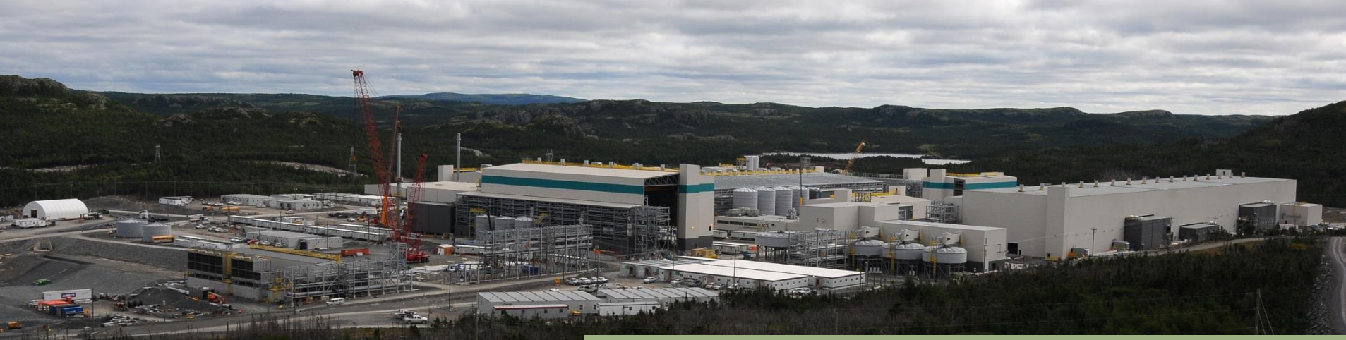
Long Harbour Development, 2012: Hydromet facility to process Voisey's Bay Ni-Cu-Co ore.
