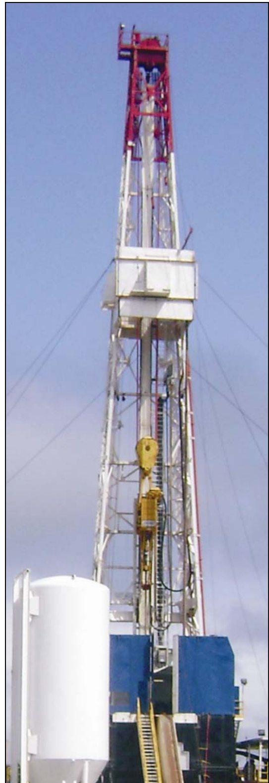
Nabors C45 drill rig at Garden Hill South
