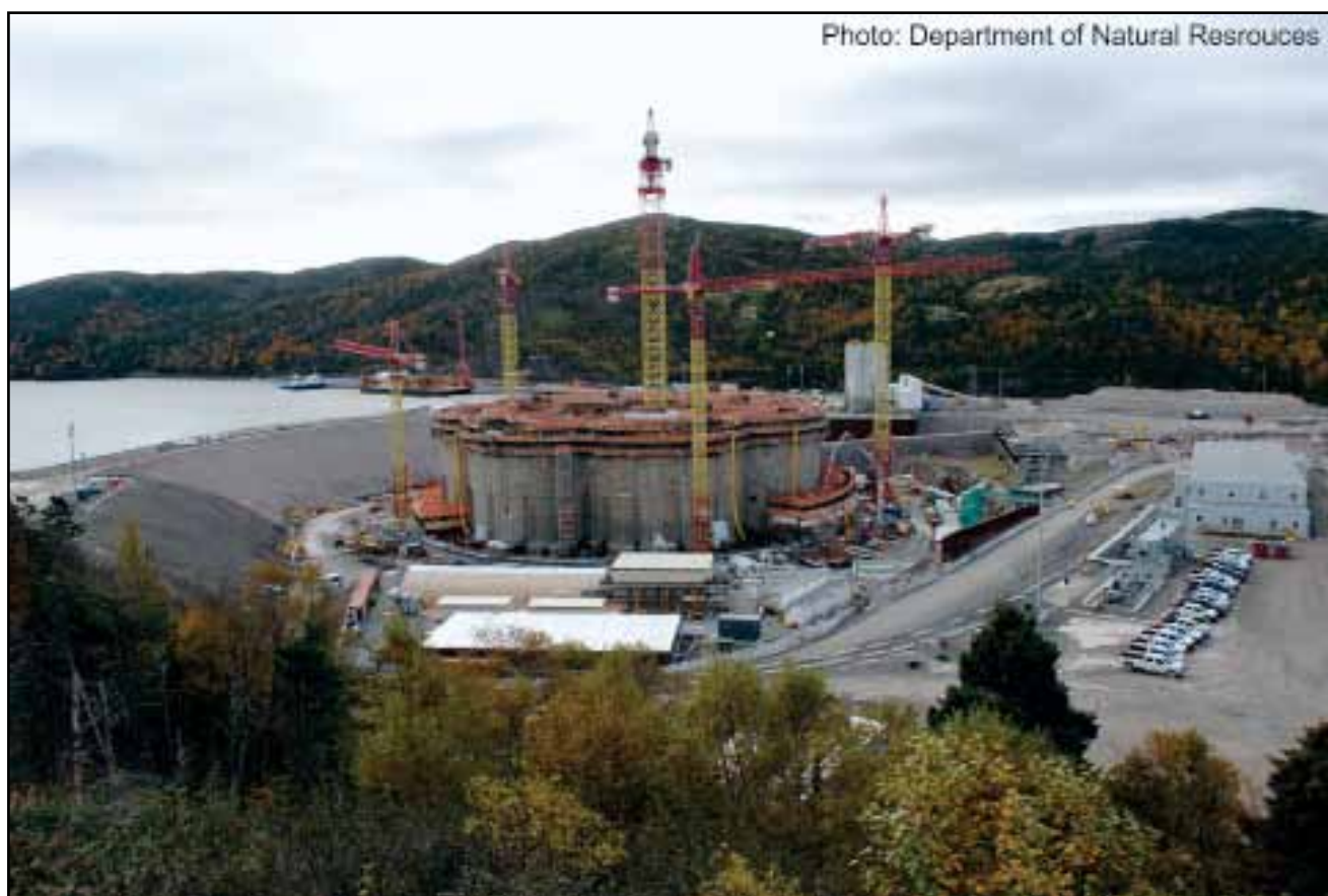
Figure 16 - Hebron GBS under construction Bull Arm fabrication site, August 2013
