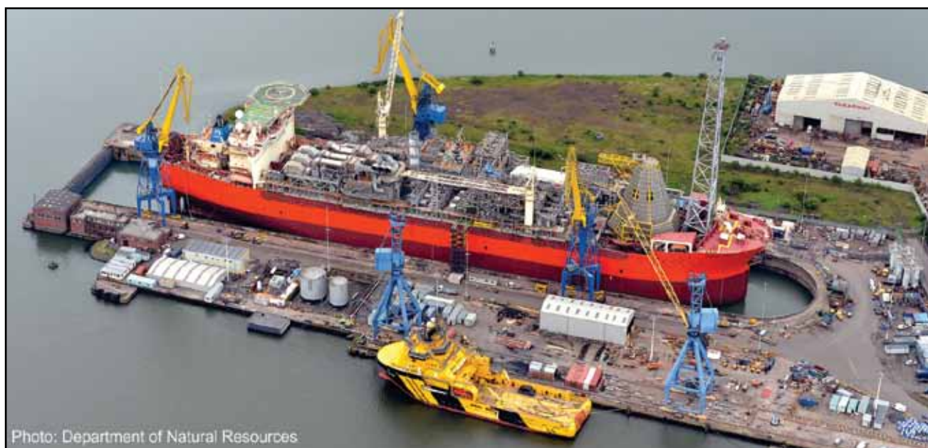
Figure 8 - White Rose FPSO SeaRose in Belfast Dry Dock
