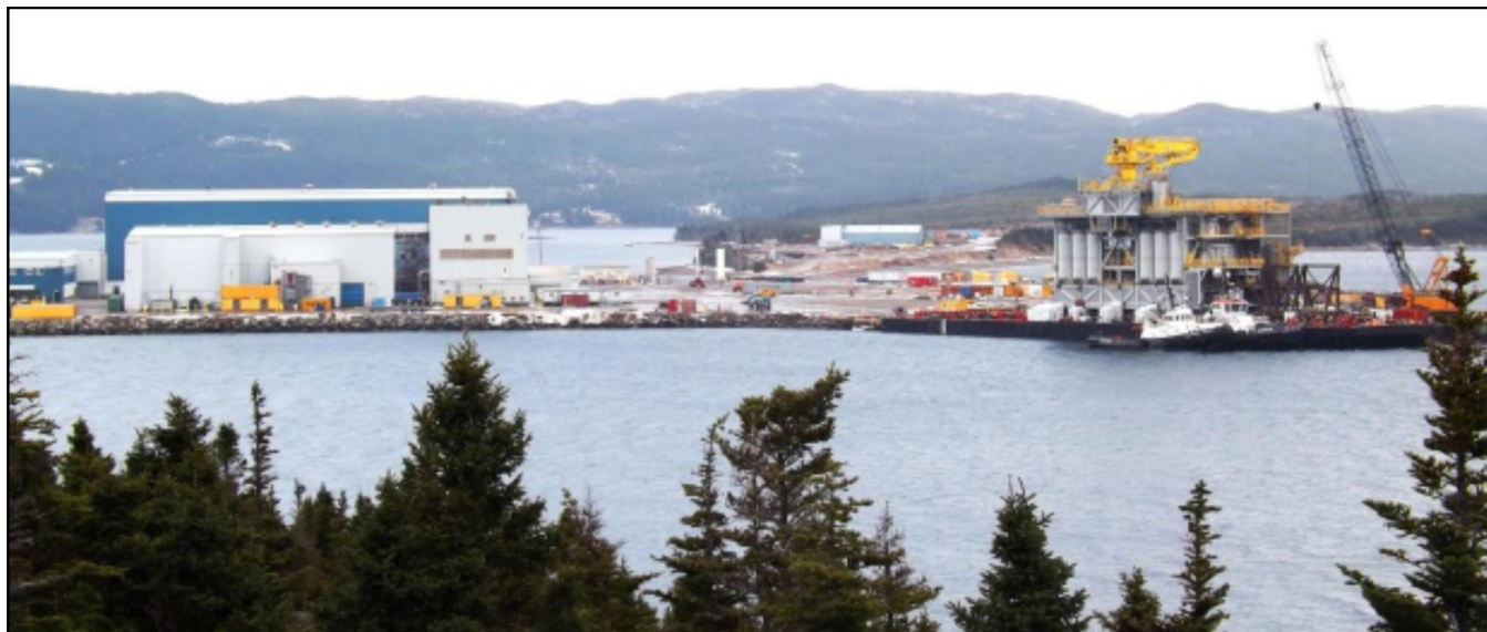
Figure 14 - Drilling Support Module for the Hebron project being fabricated at Marystown
