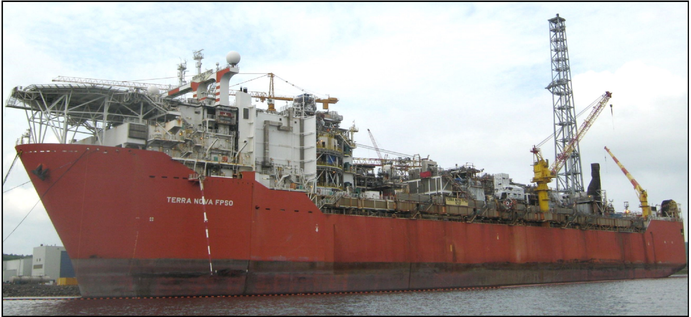
Figure 6 - Terra Nova FPSO in Marystown
