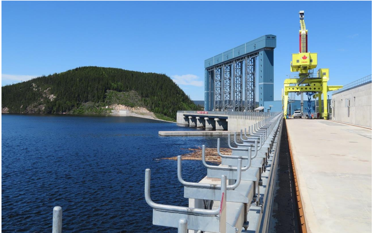
Photo 2: Muskrat Falls power intake deck and spillway with small number of woody debris pieces in front of intakes.
