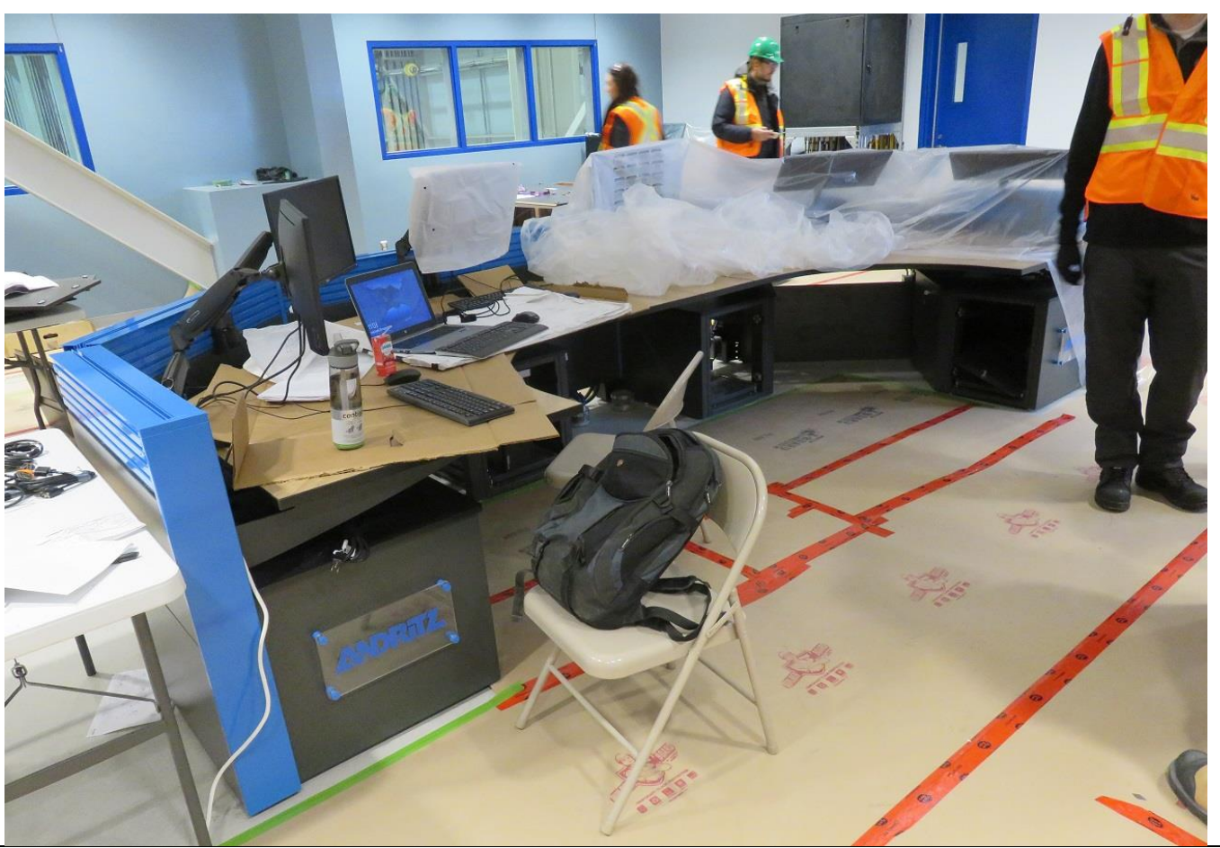
Photo 5: Control room equipment installation in progress.
