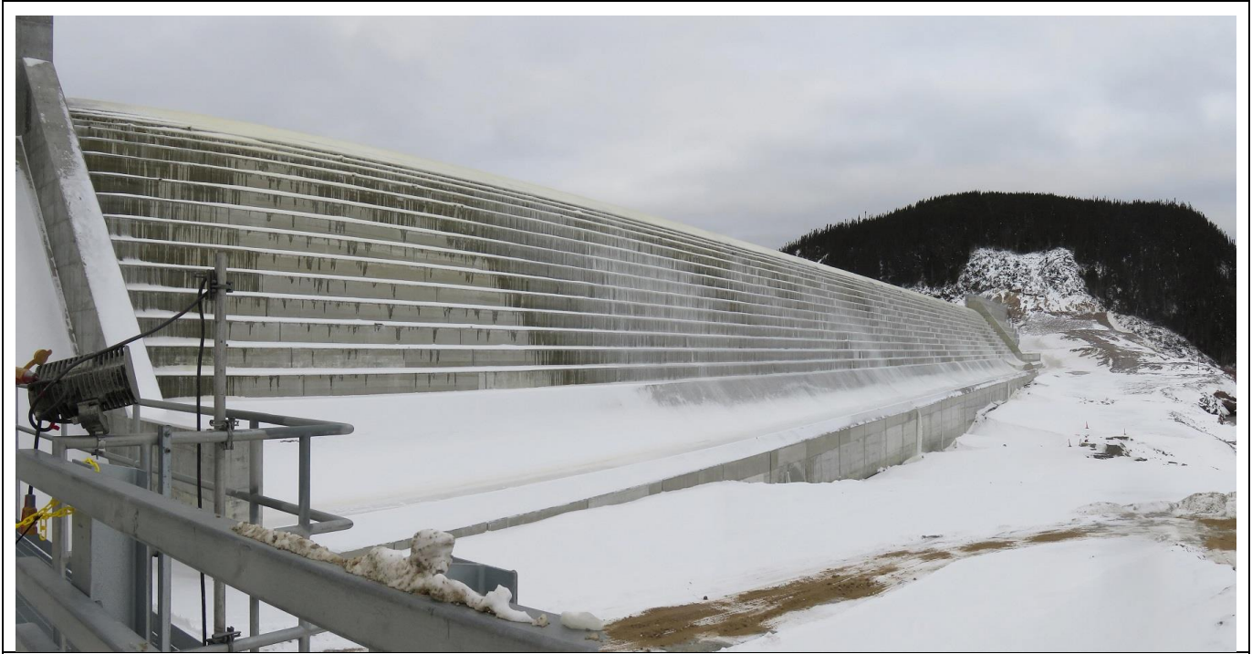
Photo 2: Downstream side of RCC dam at time of site visit – winter conditions.
