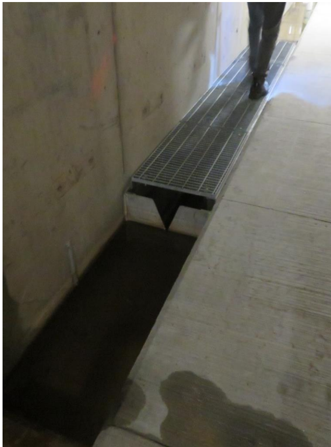
Left - Photo 7: Typical V-notch weir for measuring flow in drainage gallery ditch.
