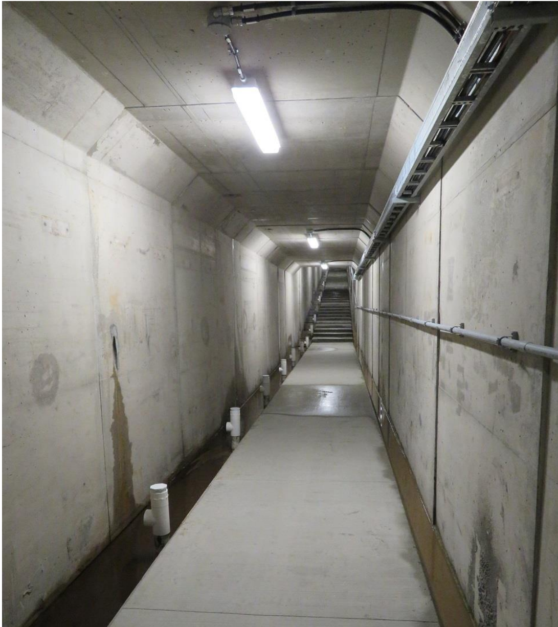
Photo 6: North Dam drainage gallery.
