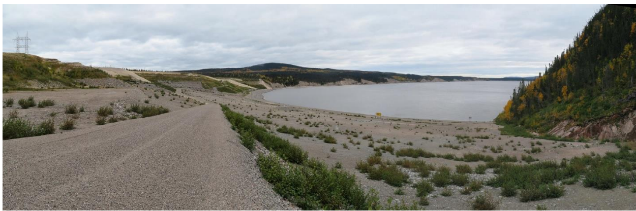
Photo 5: Downstream side of North Spur.
