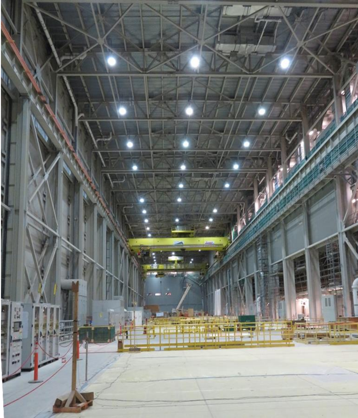
Photo 3: Muskrat Falls powerhouse interior.
