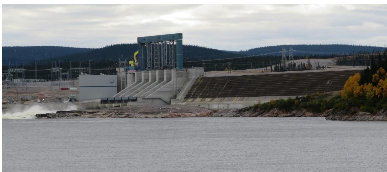
Photo 2: Muskrat Falls spillway and north dam.
