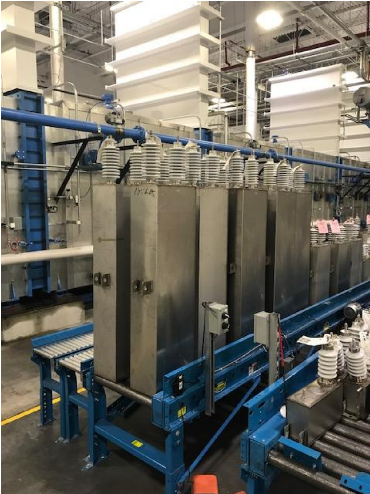
Photo 6: Drying and oil filling steps.
