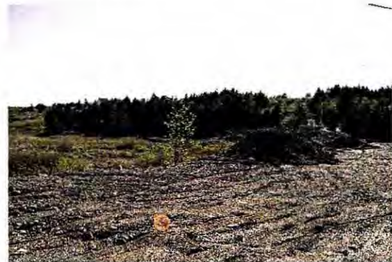
Wetland infilling on Harbour Drive.
