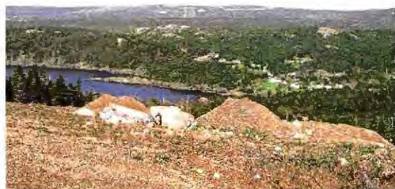
Earthworks for residential development occurring on hilltop along Cemetery Road.
