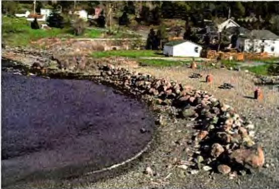
Shoreline armoring along The Tide.
