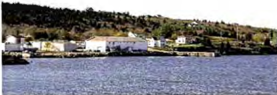
Variety Foods Ltd. Plant in Harbour Main
