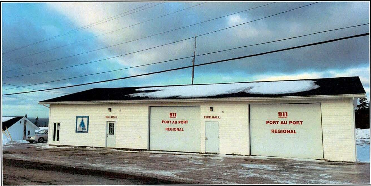
Illustration 8: Fire Hall / Town Office in the Town of Port au Port West – Aguathuna – Felix Cove
