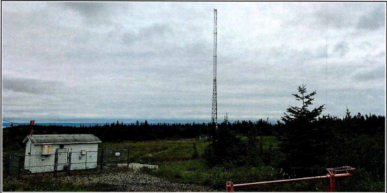
Illustration 8: Public Utility Use, Radiocommunications Lattice Tower on Father Joy's Road
