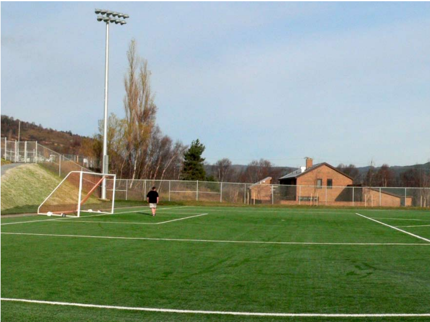
Wellington Street Sports Complex
