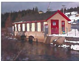
Port Union Hydro-Electric Generating Station
