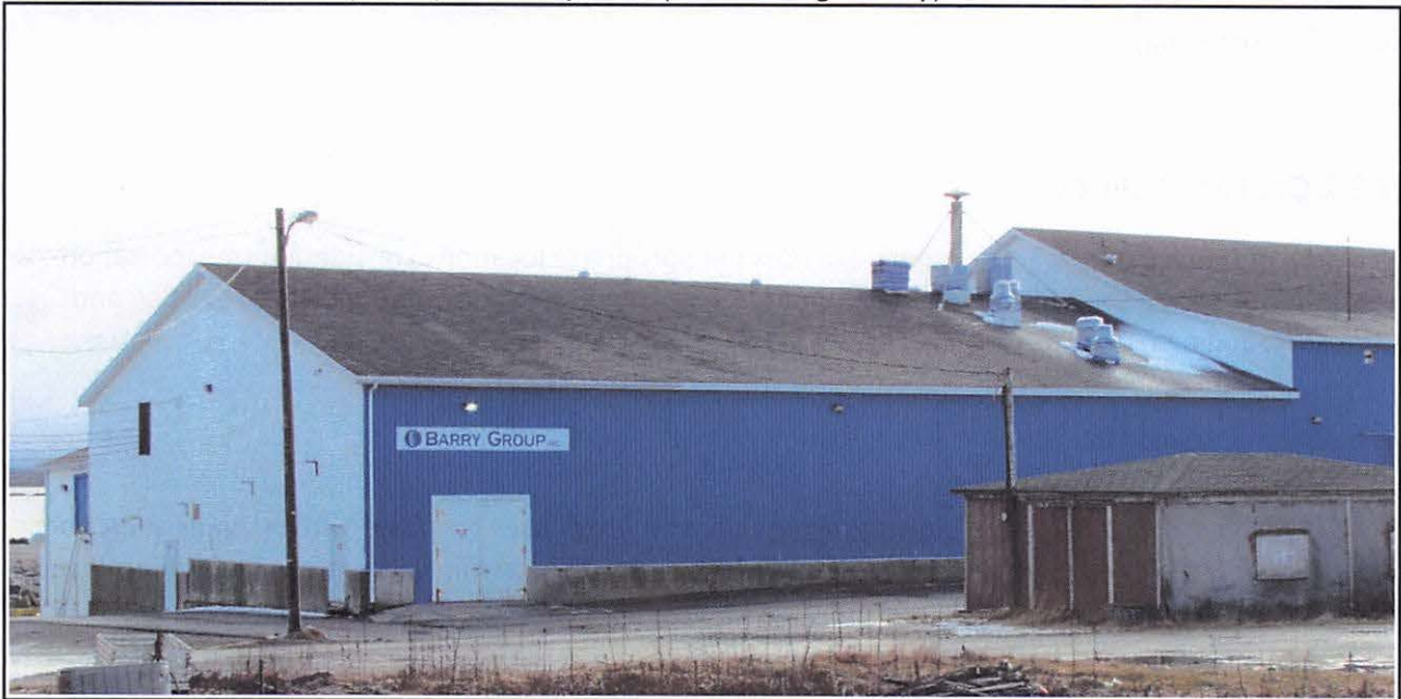
Illustration 12: Barry Group Inc. (Secondary Shrimp Processing Facility)
