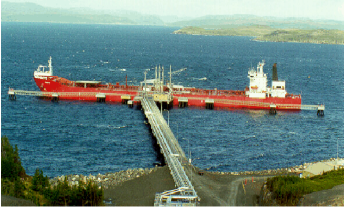
Figure 2.6 Newfoundland Transshipment Terminal Berth
