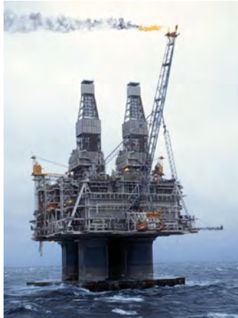
Figure 2.4 Hibernia Gravity Based Structure (GBS)
