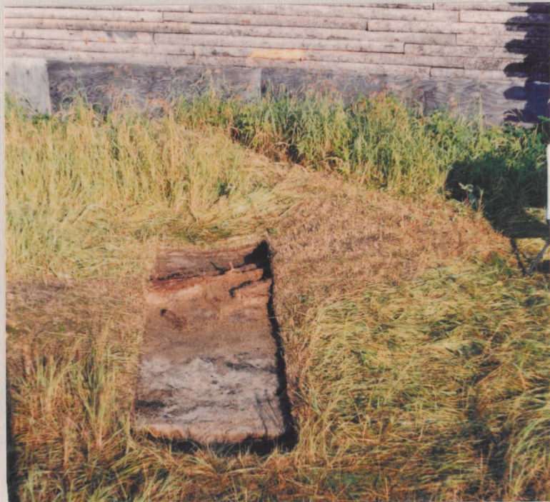
Figure 11 Ferguson Bay site; trench across the log cabin's east wall
