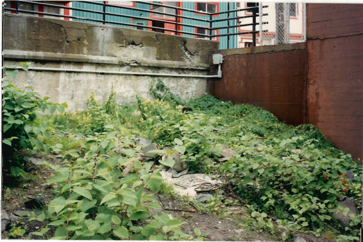
Figure 4. Backlot 296 Water Street, north east corner.
