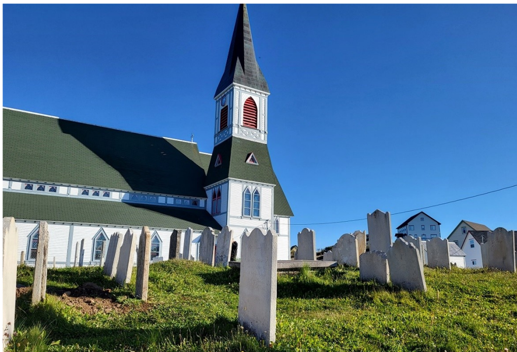
Figure 2: St. Paul's Anglican Churchyard, Trinity after our restoration.
