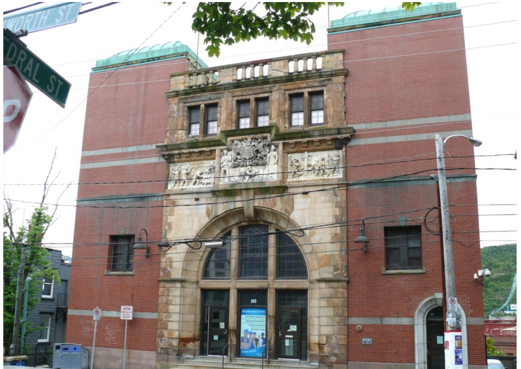
Figure 3: Former Newfoundland Museum on Duckworth Street.
