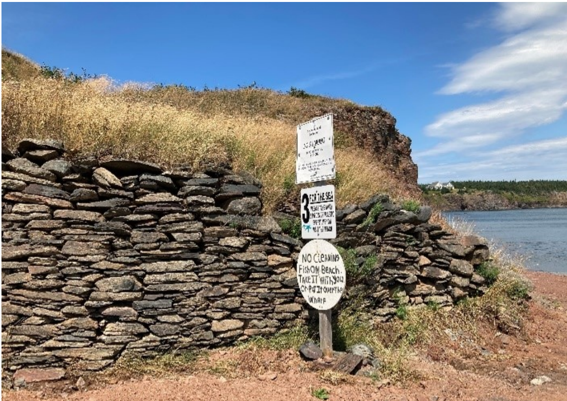
Figure 10: The dry laid stonewall used to stabilize the eroding embankment.
