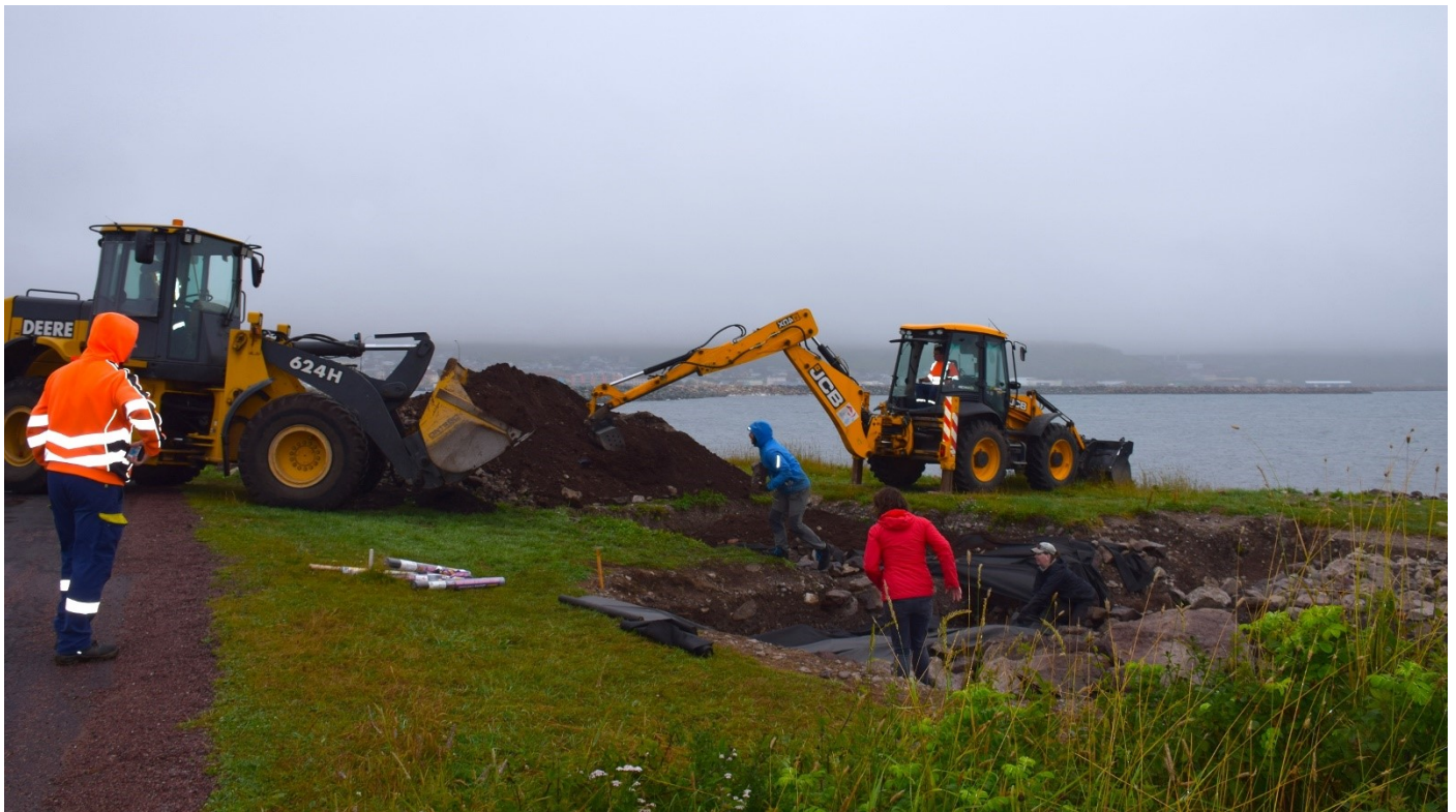
Figure 8: End of season backfilling of the Anse à Bertrand site.
