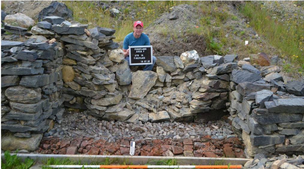
Figure 1: Collapsed back wall of the Mansion House (Structure 16) fireplace, looking south, after displaced wall rocks were removed.
