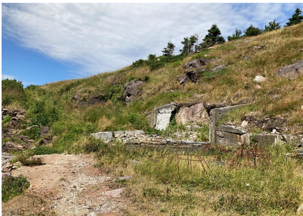
Figure 7: Remains of the Caplin Cove Wharf.
