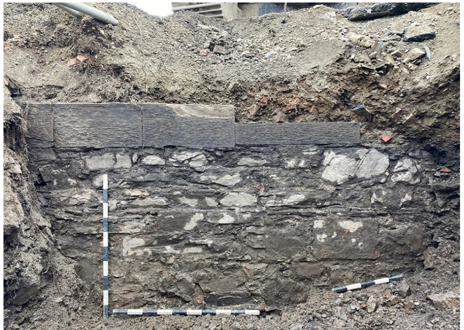
Exterior of the Custom House’s western wall. Most of the mortared stonework would have been buried during the structure’s life.
