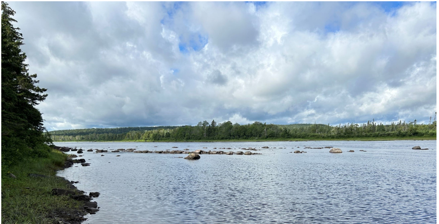
Figure 1: The rock weir, known as “the works” photographed at low tide. Caution is needed when navigating the river in this area by boat to avoid damaging propellers.
