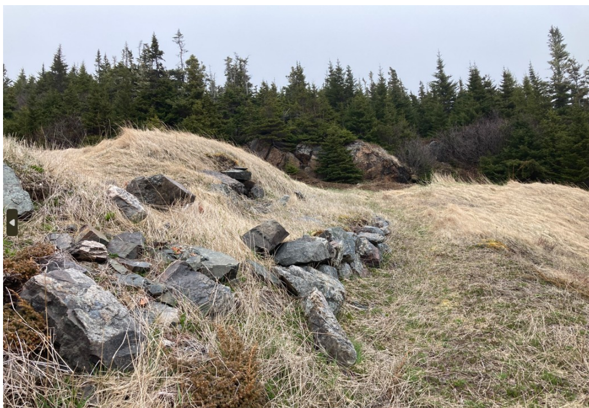
25.02 Figure 4: Stone retaining wall feature (at centre, Jobs Head ) separating the path down to the beach from a cellar pit, above.
