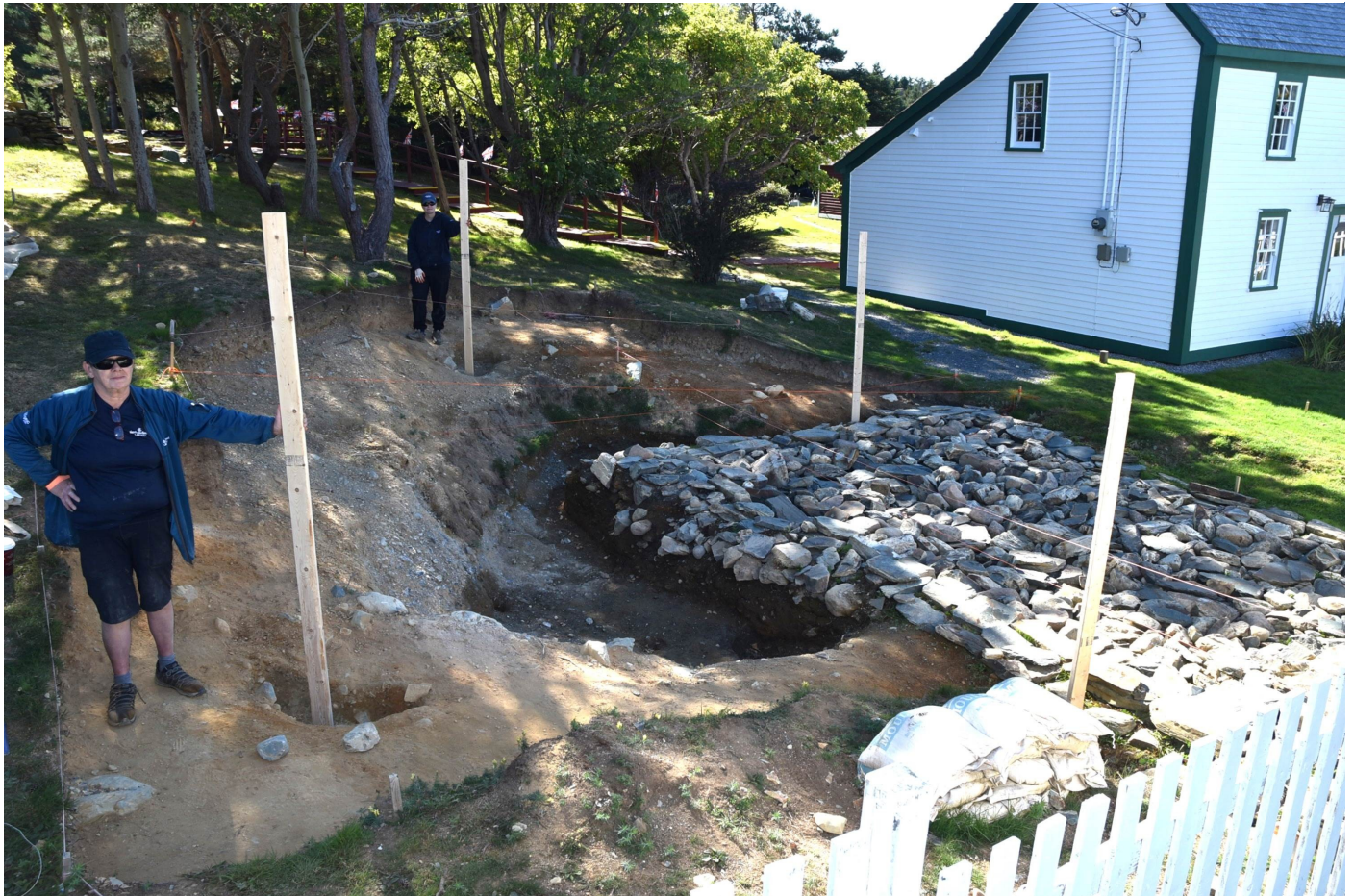
Figure 7: The sawpit with posts marking the four corners of the sawpit house.
