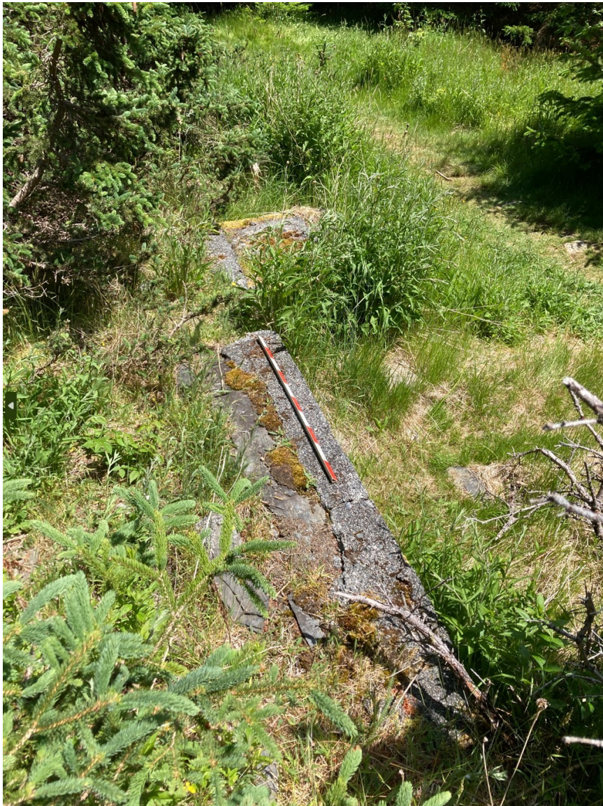
25.10 Figure 1: A concrete foundation on the East Coast Trail at ChAf-03.
