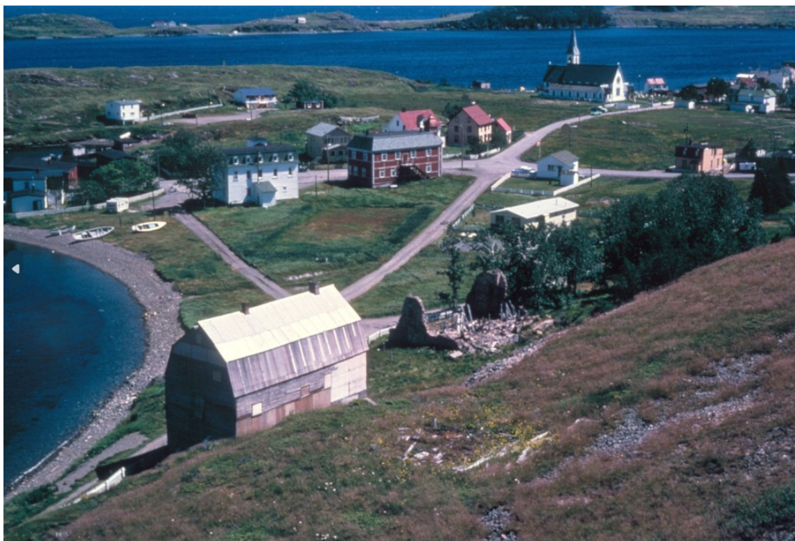
25.02 Figure 1: Photo from 1978, showing the Ryan's Store/ Mercantile Premises structure. Note the absence of an extension, though signs of its previous existence are visible on the structure. The ruins of the Lester-Garland building are to its right (PAO 1978 00-0006).
