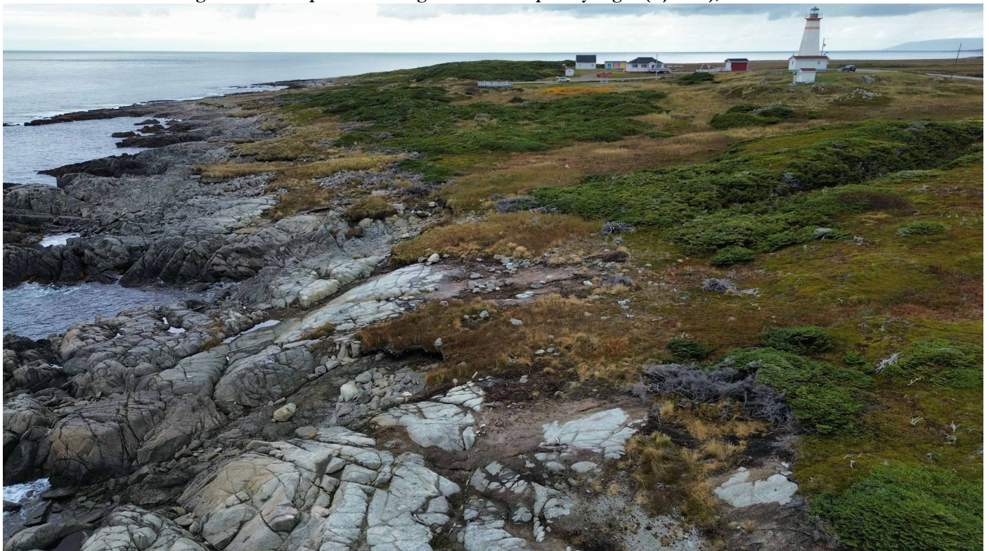
Figure 9: Drone photo showing erosion at Cape Ray Light (CjBt-01), view west.
