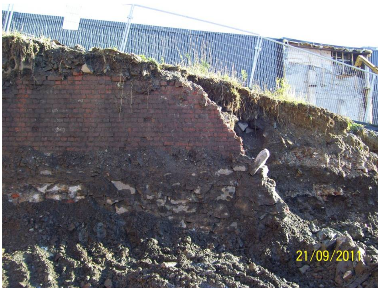
Figure 2 Exposure of a remnant brick wall, resting on an earlier stone foundation wall, Woolworth's site.
