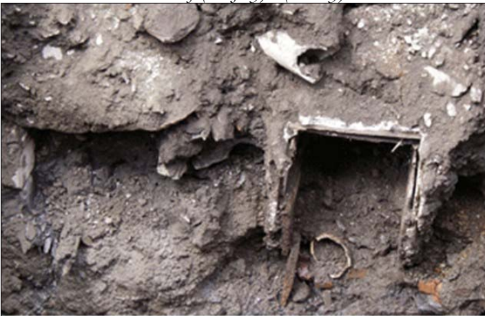
Some of the maze of stone connecting sewers, Water near Holloway Street. The sewer at left is of stone, and can be seen to take in ceramic drains from surrounding former structures. At right, a concrete sewer of more recent construction (14 Aug). (Penney)
