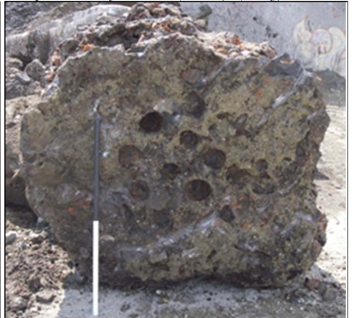
Pits in the base of the pile cap indicate that it was created directly on wooden piles (14 Aug). (Penney)
