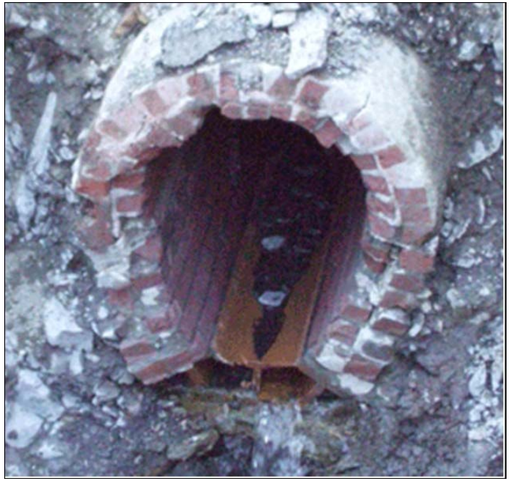
Ovoid double-lined brick sewer, presumed to date from 1893, showing the ceramic trough and underlying channel (24 Aug). (Penney)
