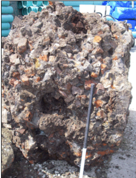
A portion of a brick/ amalgam pile cap, at Jobs Cove. It is posited that rubble was used to "make ground" after the 1892 fire by sprinkling dry cement on it in layers much as salt is spread on fish in salt bulk (14 Aug). (Penney)
