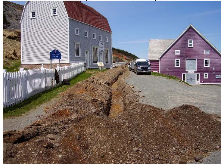
The trench dug for electrical services from the Lester-Garland House to a recently constructed cooperage. (Skanes)
