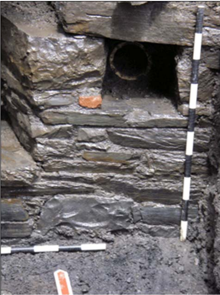
Sewer/drain tie-ins at Queens Cove, possibly associated with old Gambier Street and/or the harbour masters office etc. at the Kings Wharf (30 July). (Penney)
