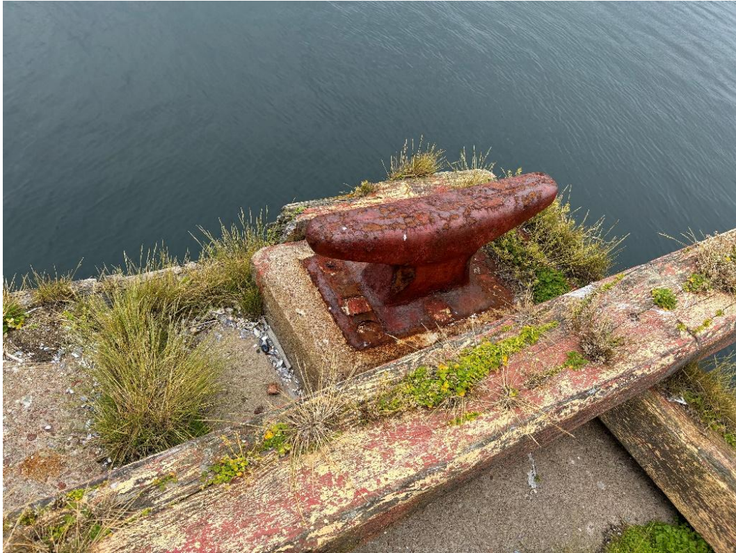
Figure 9 – Cleat on northwest corner with wheel guard detached in area.
