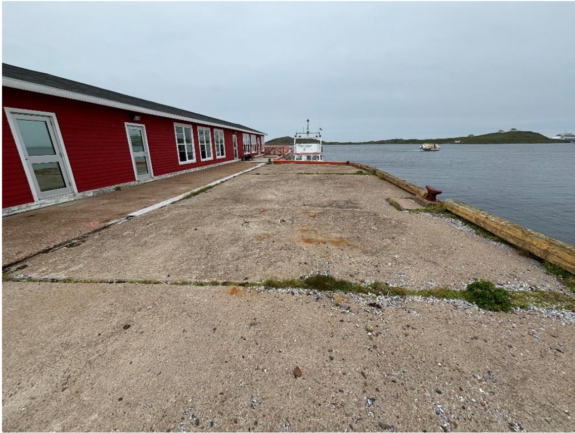
Figure 3 - Standing on northwest corner looking south.
