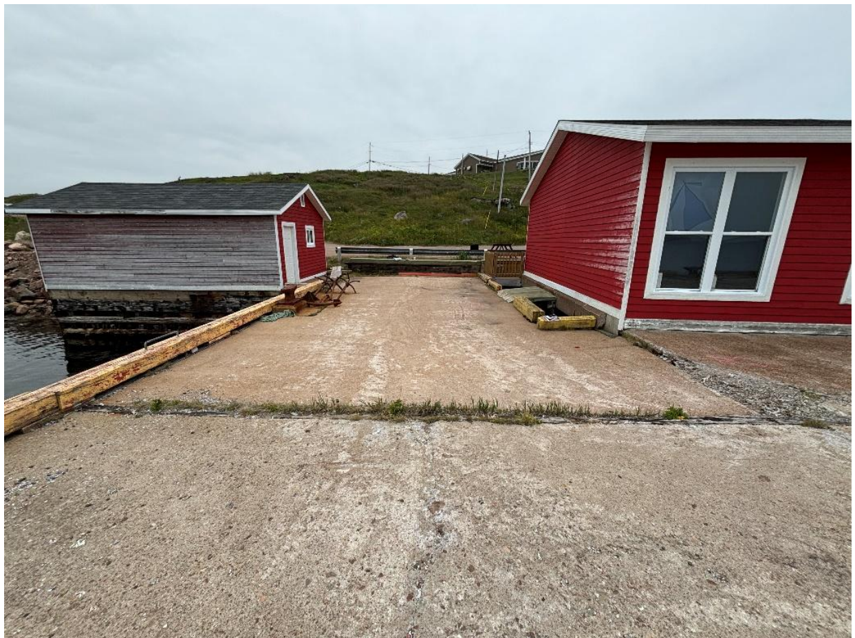
Figure 2 – Standing on northwest corner looking east (approach).
