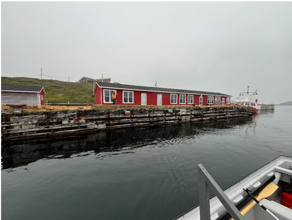
Figure 4 – West berthing face.
