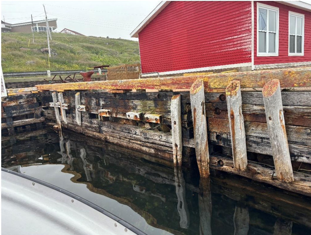
Figure 10 - North face of wharf.
