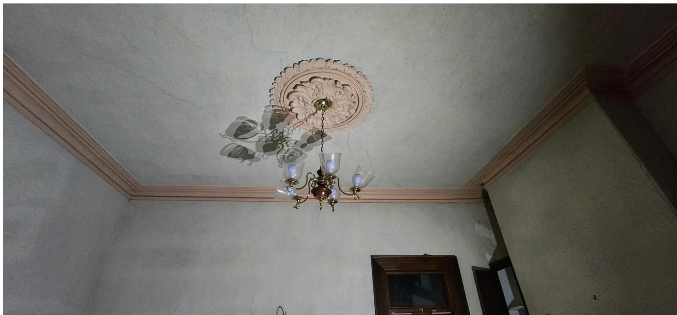
Photo 21: Ceiling medallion Room 103 looking south
