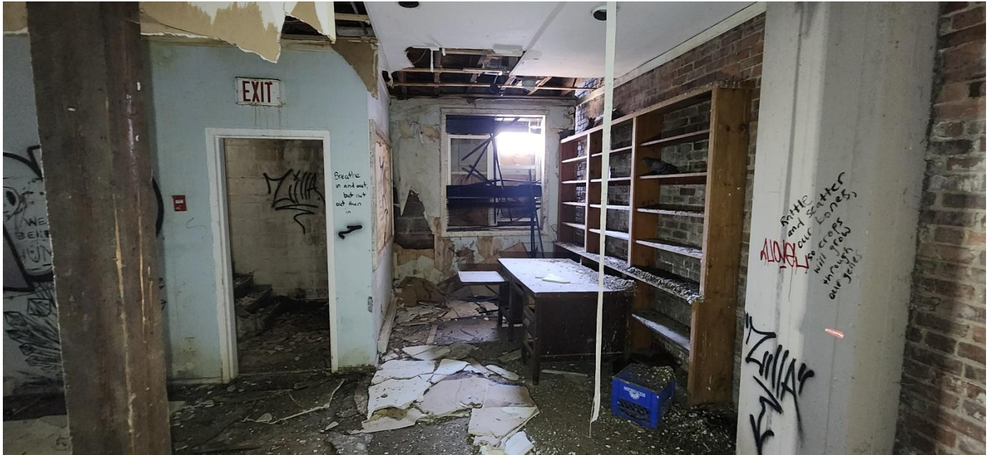
Photo 27: Room 205 looking west
