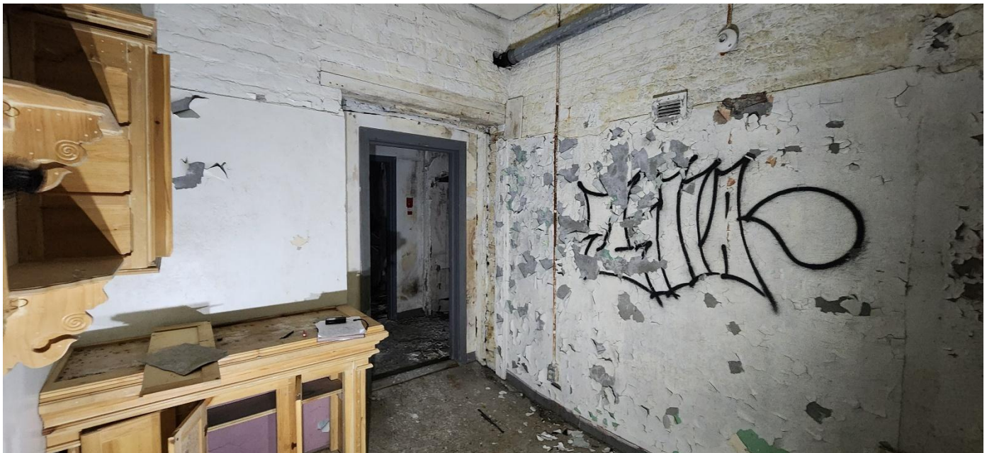
Photo 17: Kitchen 106 looking west towards tunnel
