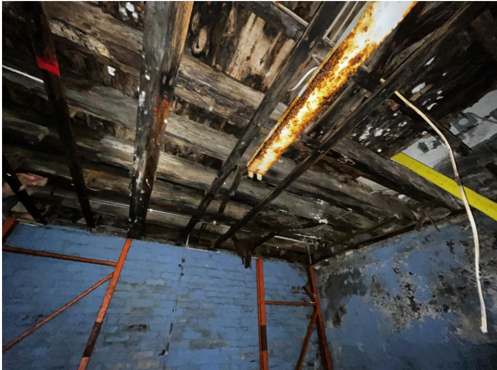
Photo 37: 106 Kitchen Floor Framing (from B03 Basement Storage)
