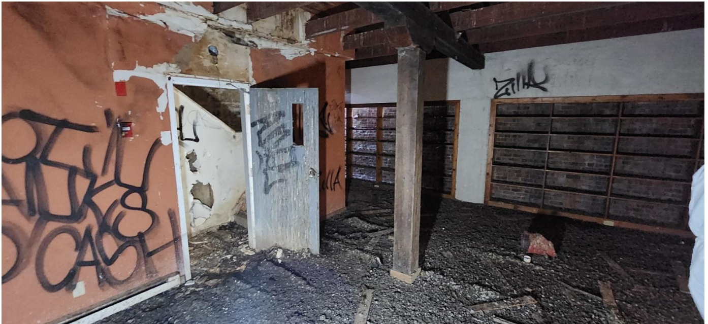
Photo 28: Room 305 looking northwest
