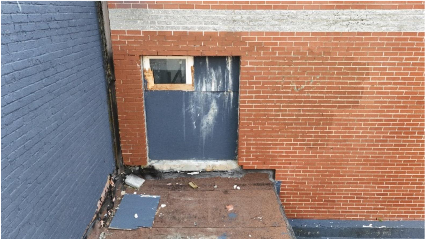
Photo 8: Partial west elevation above tunnel at level 2
