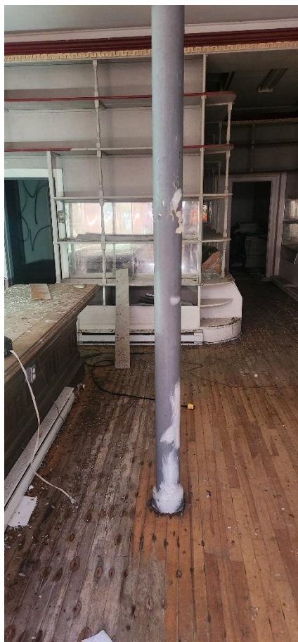
Photo 19: Round column in 102 Storefront
