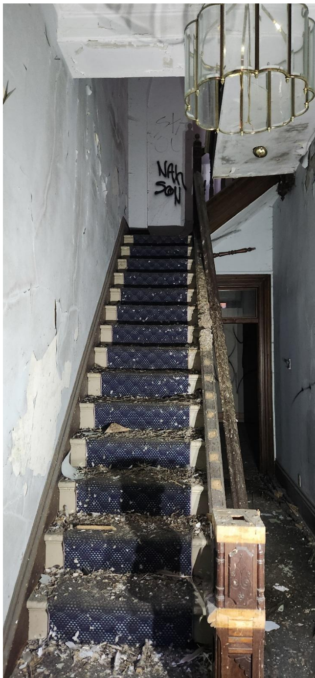
Photo 20: Stair 1 from level 1 looking north
