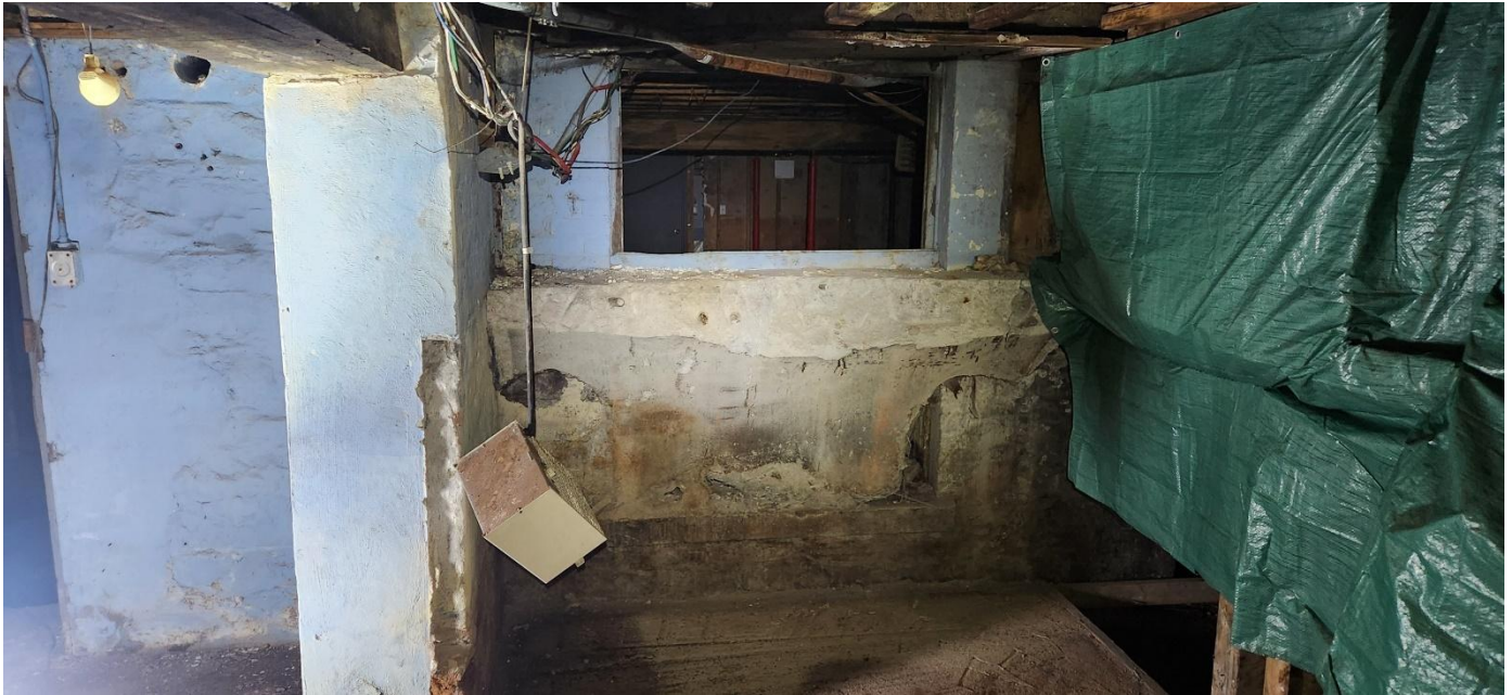
Photo 16: Basement B04 looking south
