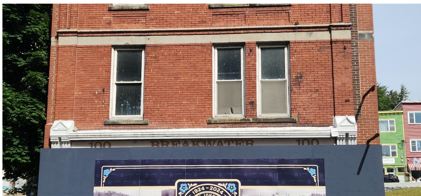
Photo 6: Partial south elevation at level 2
