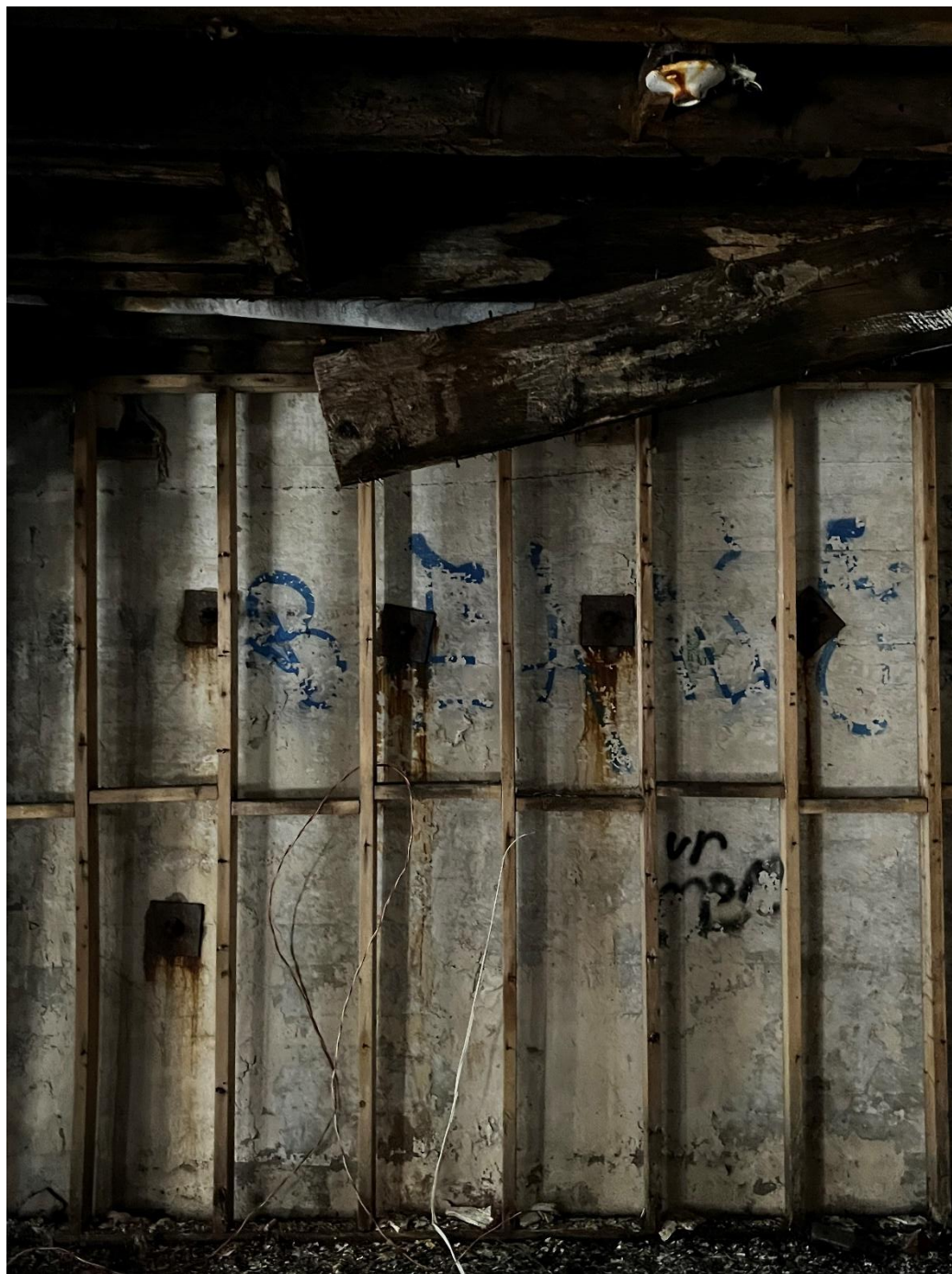
Photo 37: Concrete wall with anchors along Holloway Street
