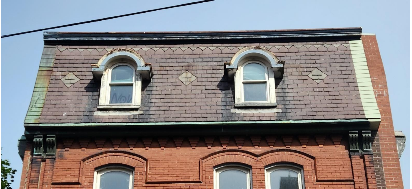
Photo 4: Mansard roof and hooded dormers
