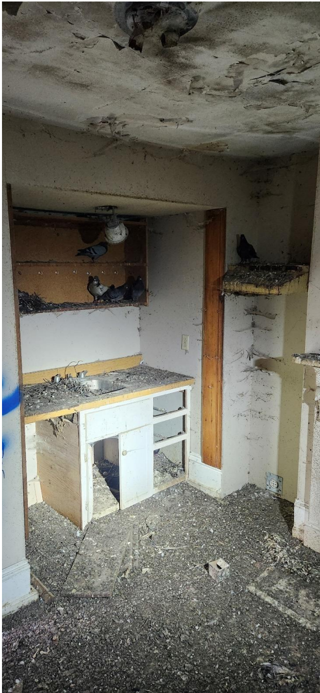
Photo 35: Room 403 looking southwest
