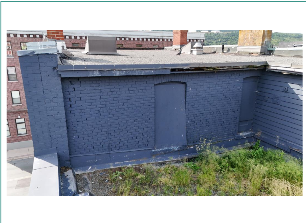
Photo 52: Partial North Elevation at Level 4
