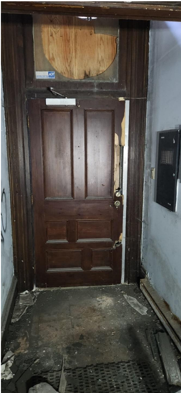
Photo 13: Inside of front vestibule entrance door
