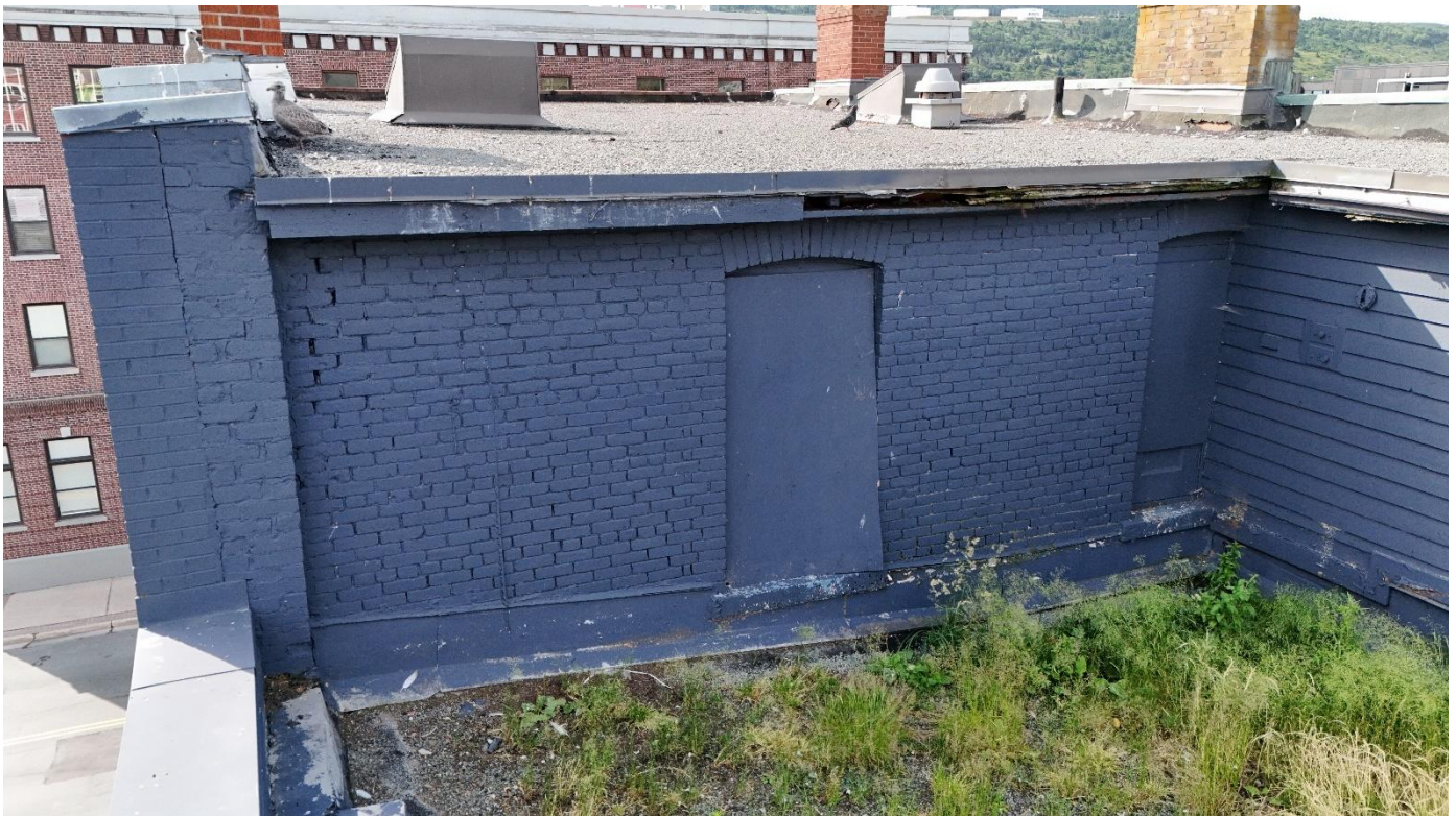
Photo 7: Partial north elevation at level 4
