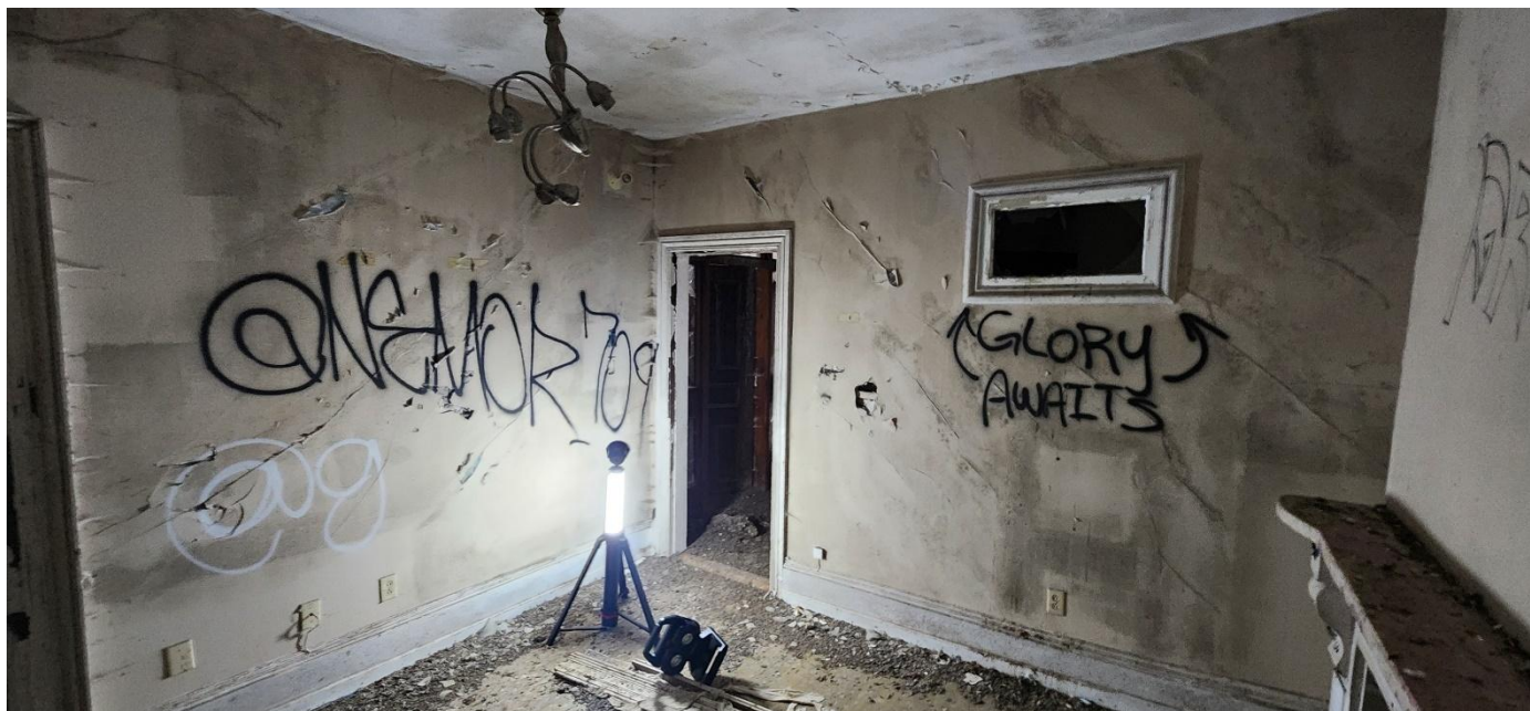
Photo 29: Room 303 looking southwest
