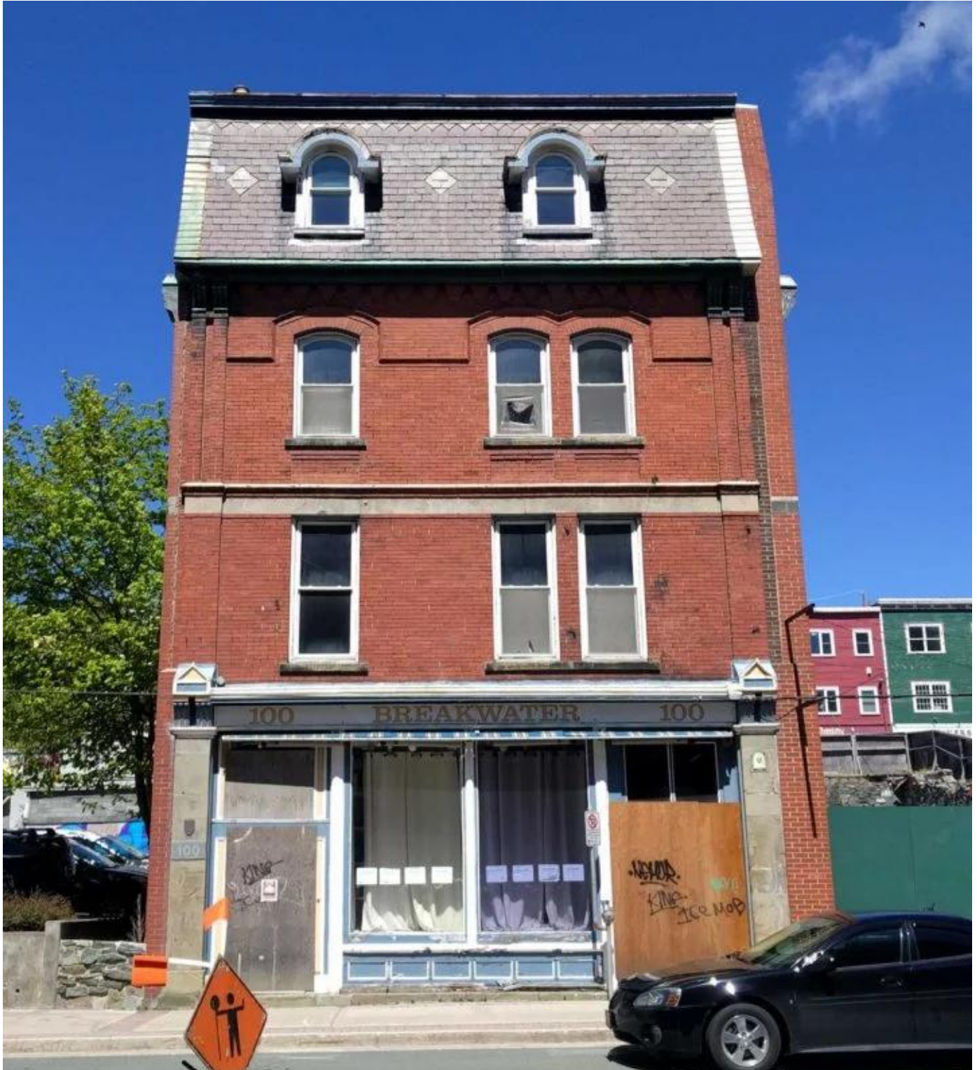
Photo 12: South elevation depicting windows and doors, and uncovered storefront, date unknown (NL Heritage)
