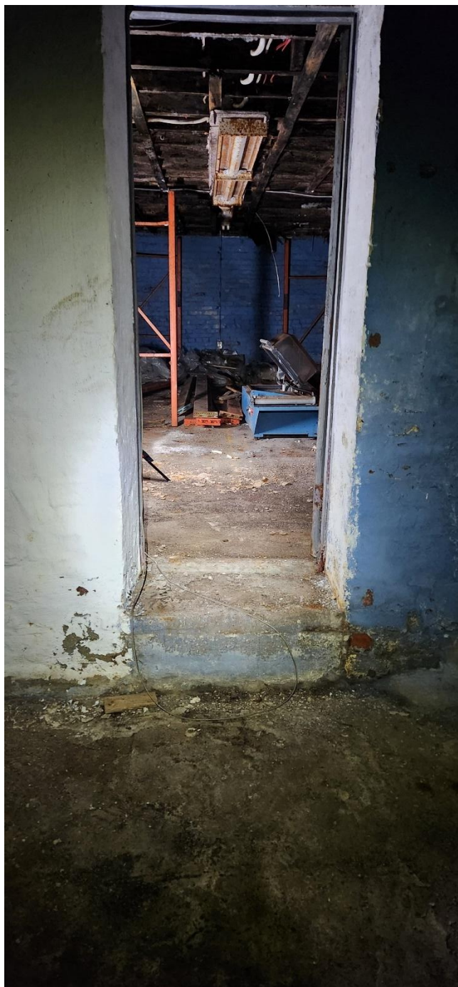
Photo 15: View into basement storage B03 looking north
