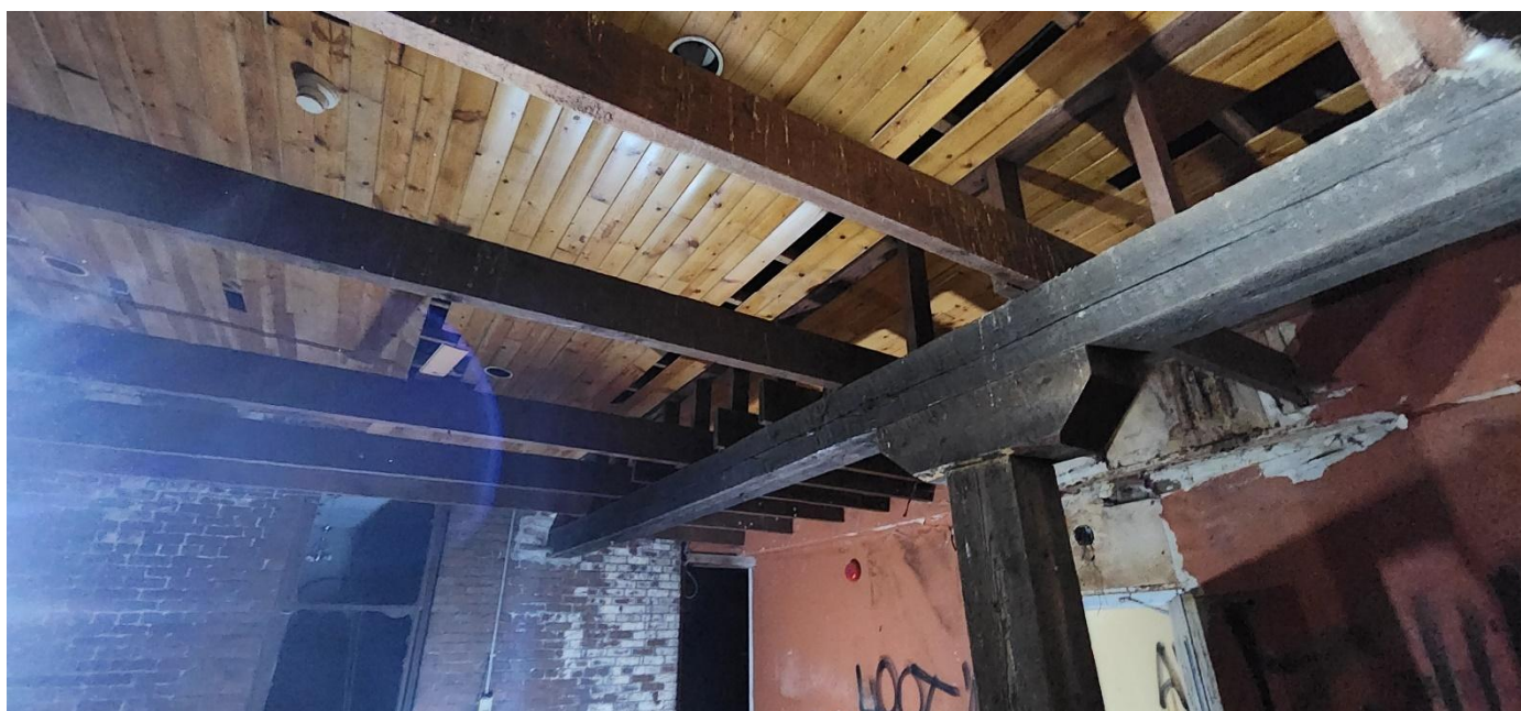
Photo 30: Room 305 looking south
