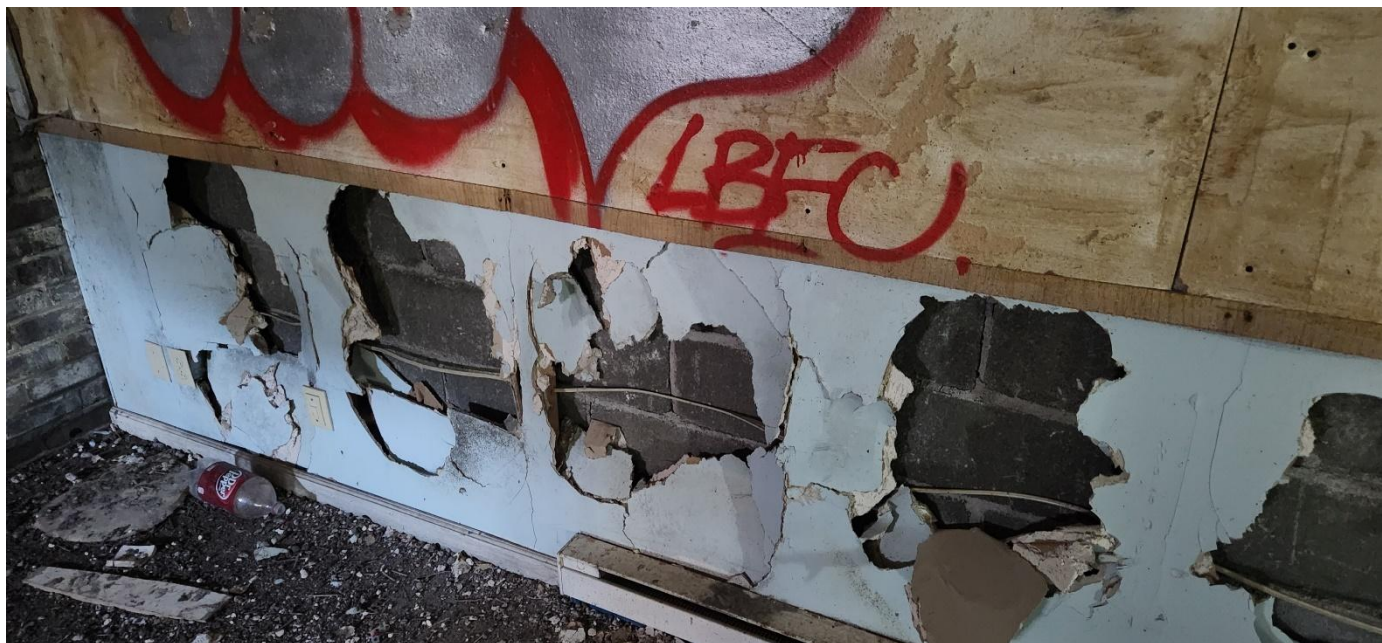
Photo 24: Room 205 looking east
