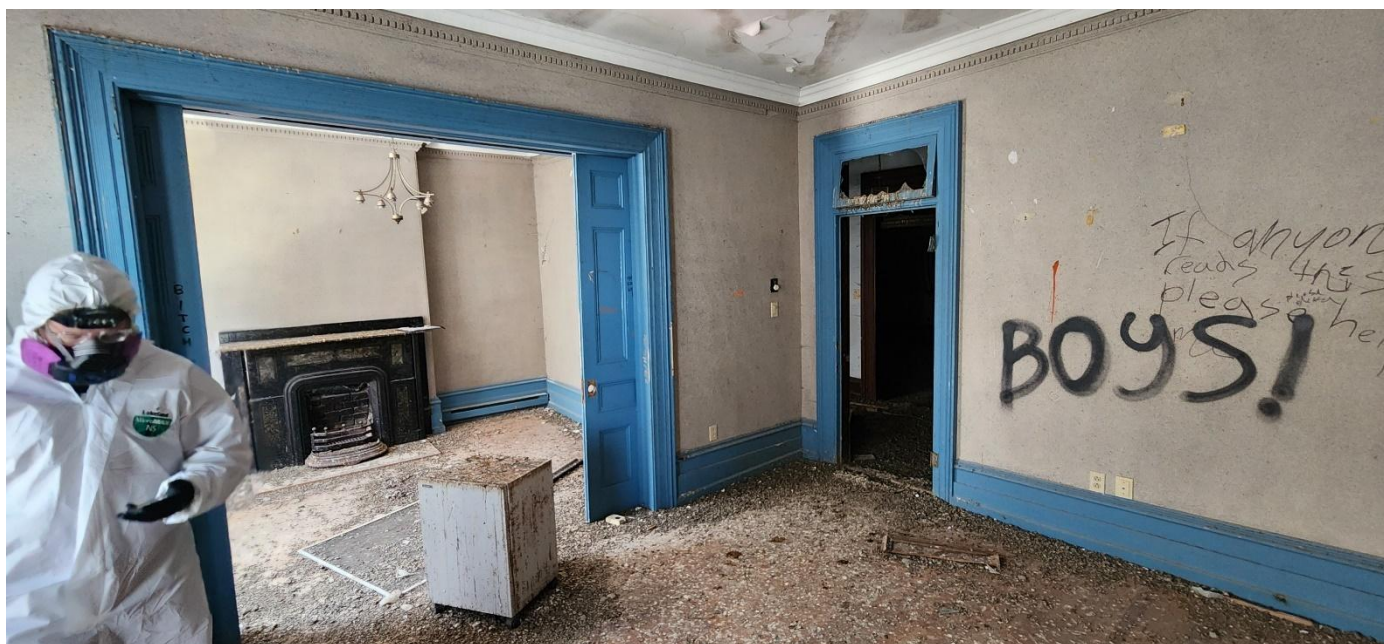
Photo 26: View from Room 202 looking west to Room 201
