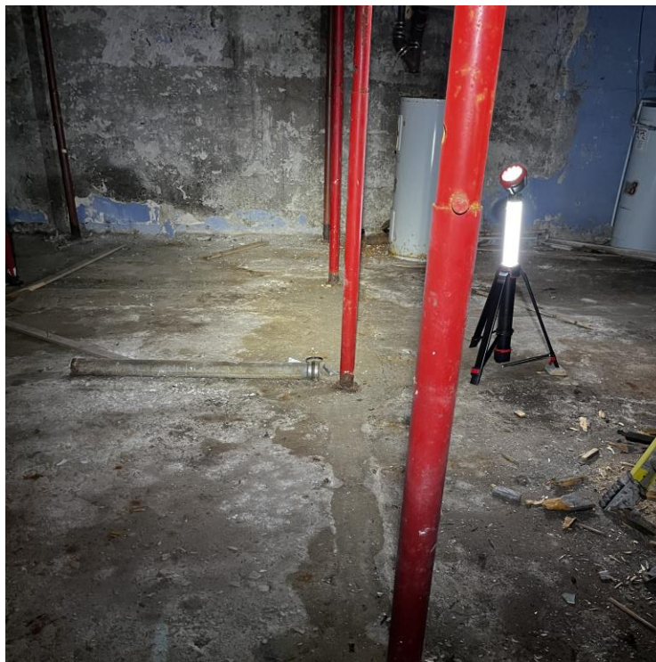
Photo 26: B01 Open Basement
