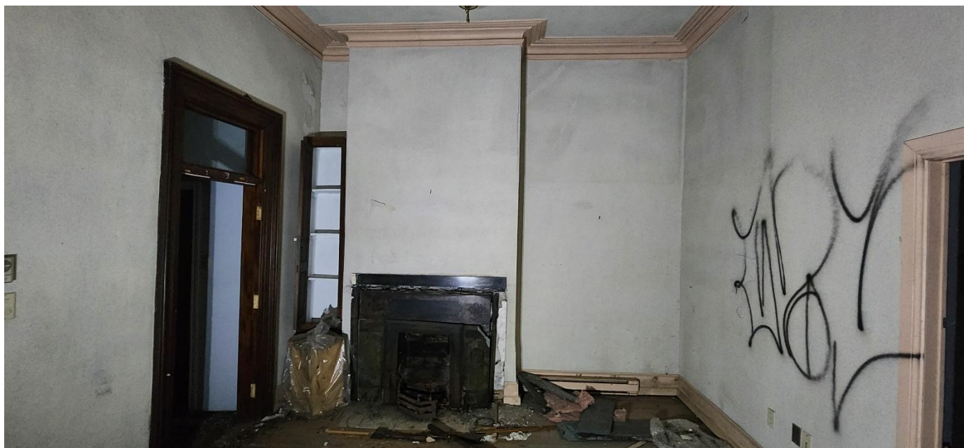
Photo 22: Room 103 looking west
