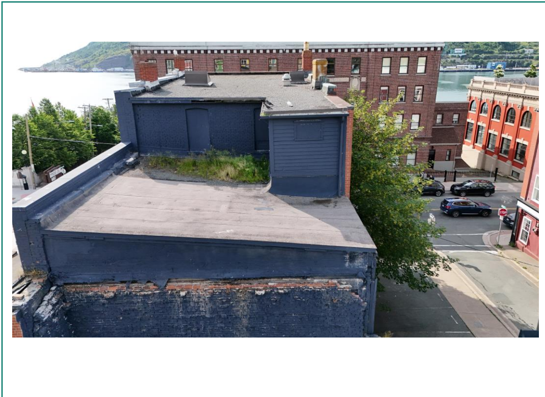
Photo 53: Partial North Elevation
