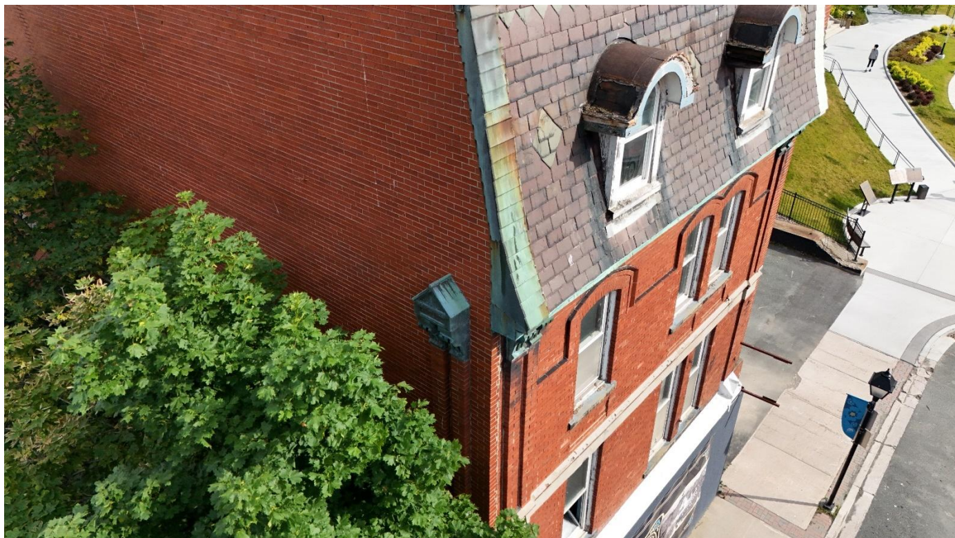
Photo 10: Aerial photo of southwest corner showing pilaster capital
