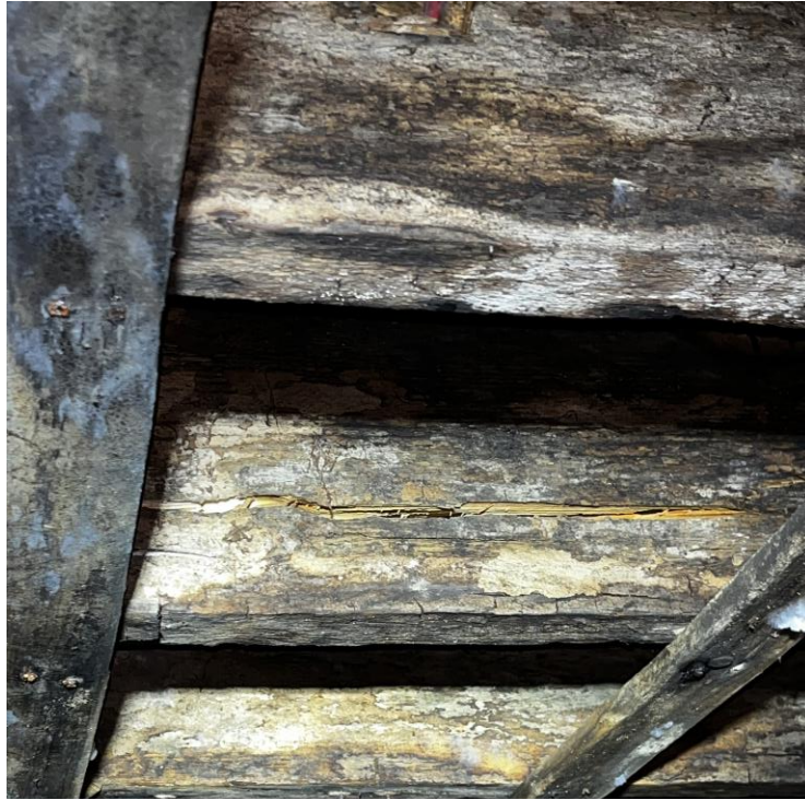
Photo 35: 106 Kitchen Floor Framing (from B03 Basement Storage)
