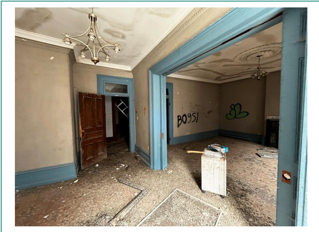
Photo 11: 201 Room and 202 Room (from 201)
