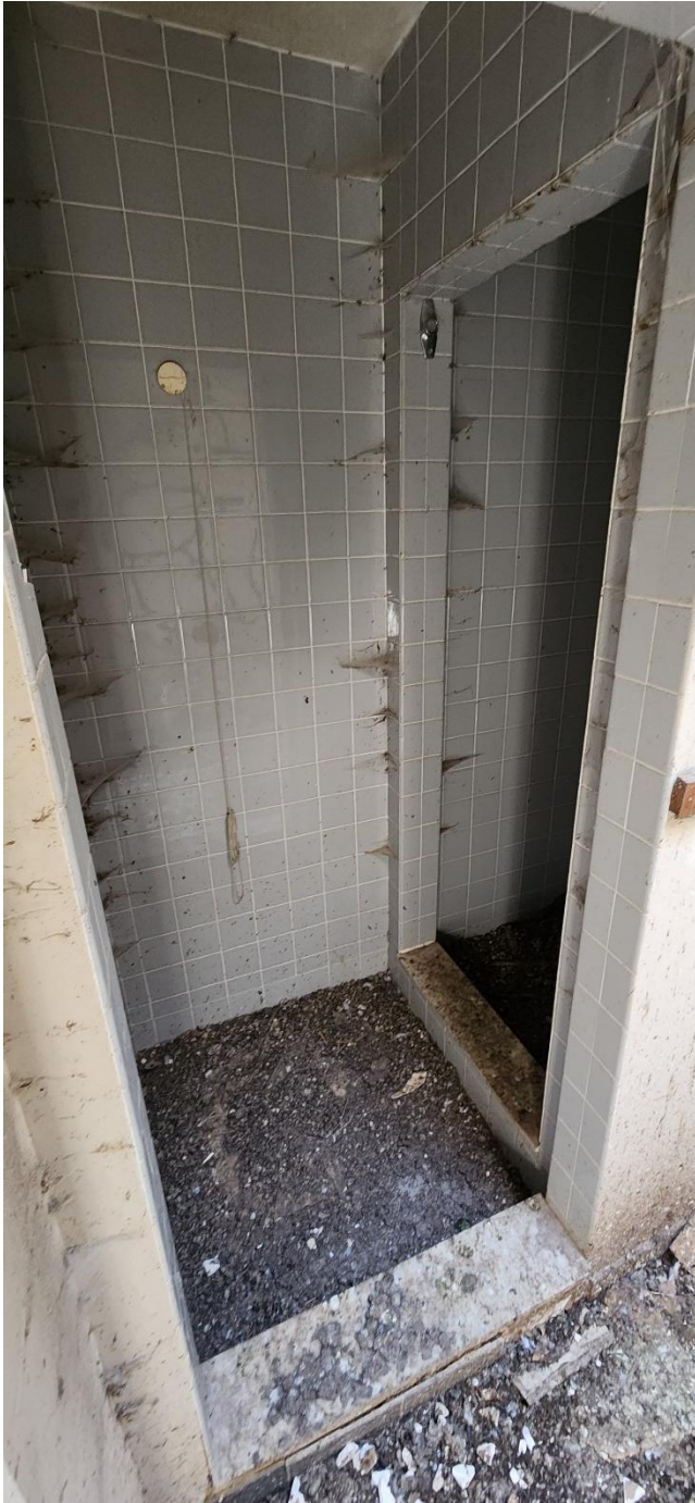
Photo 34: Room 406 looking south
