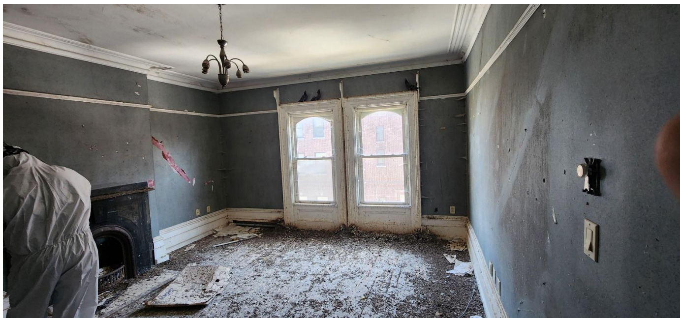
Photo 31: Room 402 looking south
