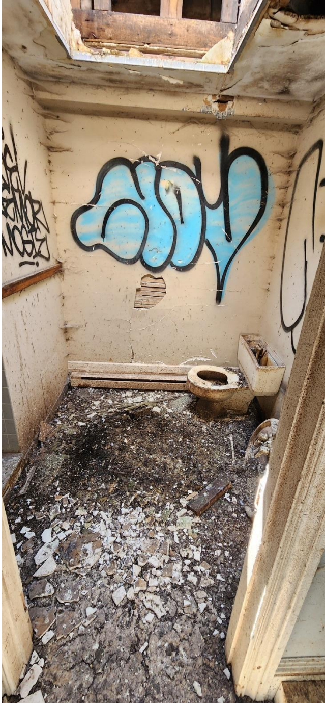
Photo 32: Room 407 looking west
