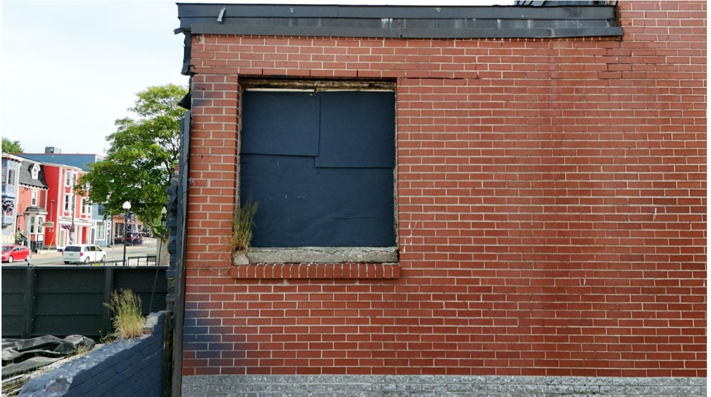
Photo 9: Partial west elevation above tunnel at level 3
