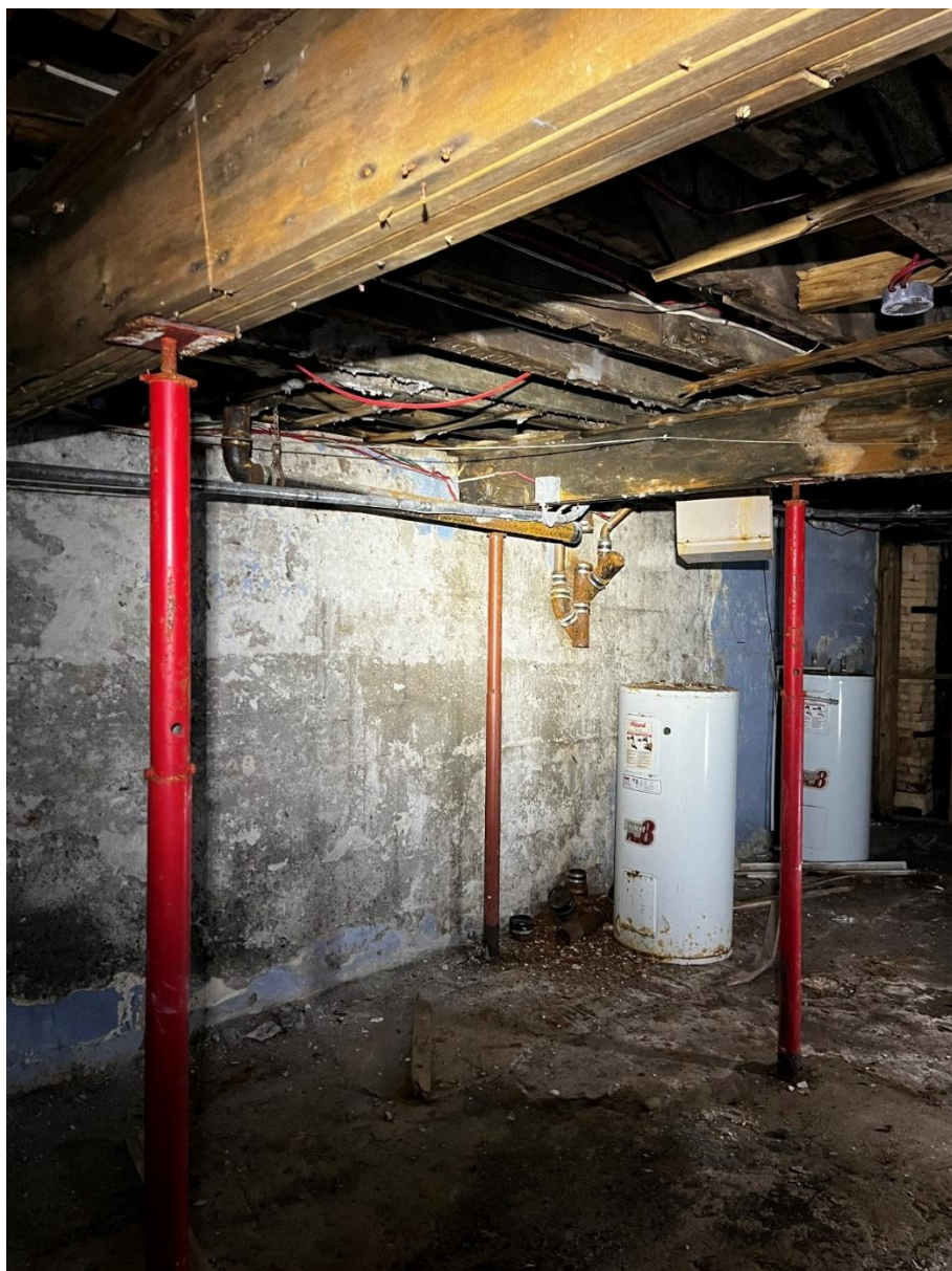
Photo 40: Level 1 floor framing Area 1
