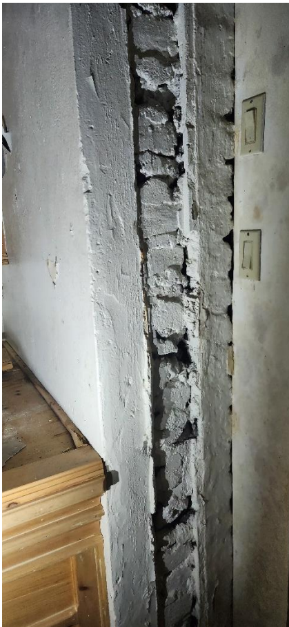
Photo 18: Wall assembly at Kitchen 106
