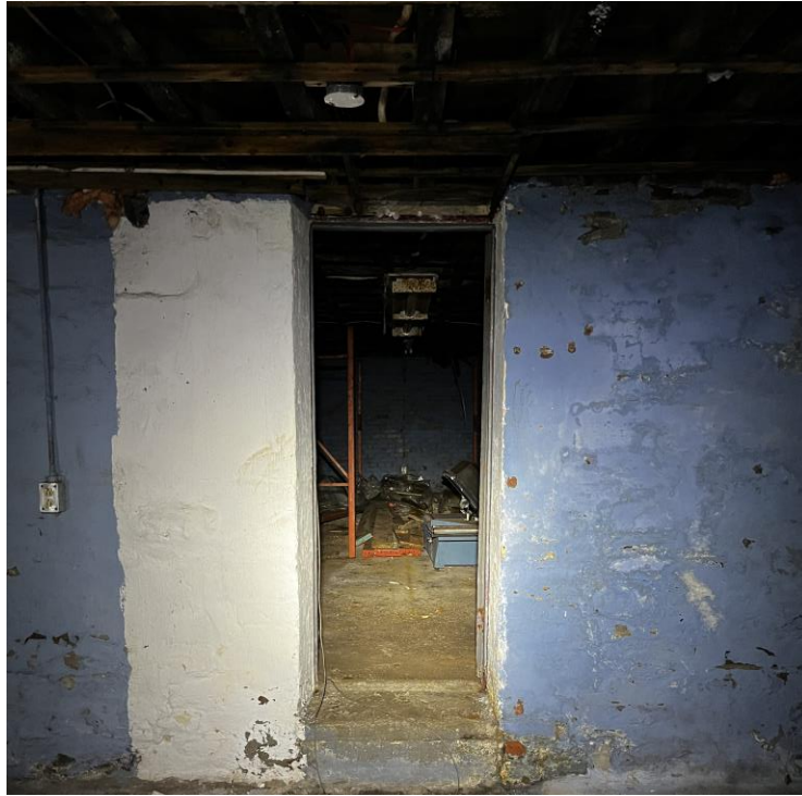
Photo 27: B01 Open Basement
