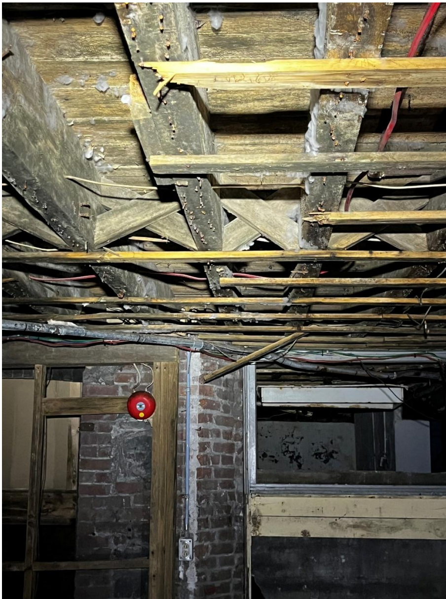
Photo 39: Level 1 floor framing Area 1
