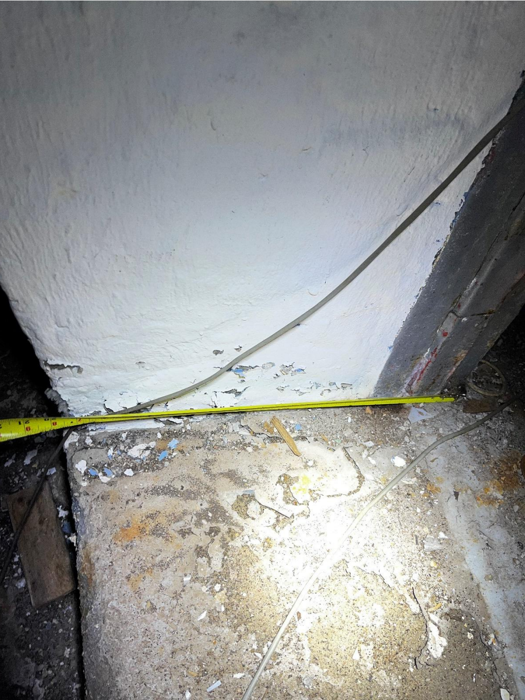
Photo 38: Old exterior wall in basement along demarcation of Area 1 and Area 2
