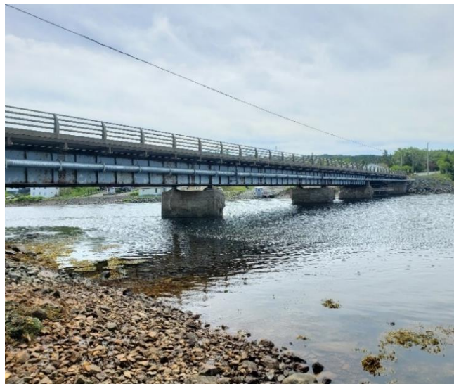
Figure 1-2: Marystown Harbour Bridge
