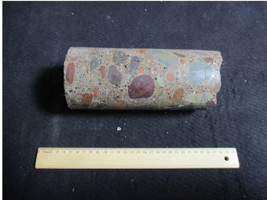
Core 14 Sampled from South Abutment - Foundation. Near Ground Level
