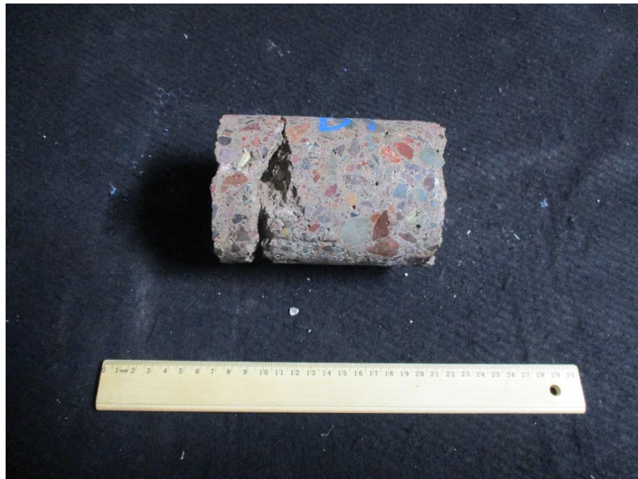
Core D1 Sampled from Bridge Deck
