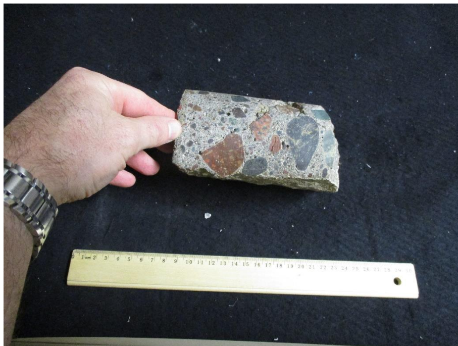
Core 33 Sampled from Swing Pier – Vertical face
