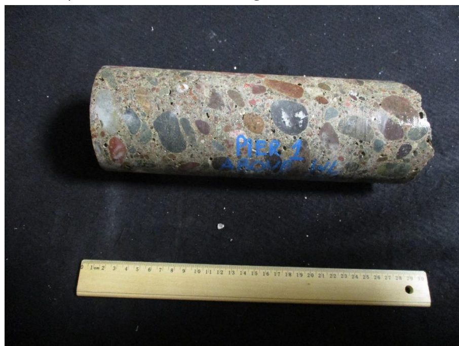
Core 27 Sampled from Pier 1 – Above high-water line
