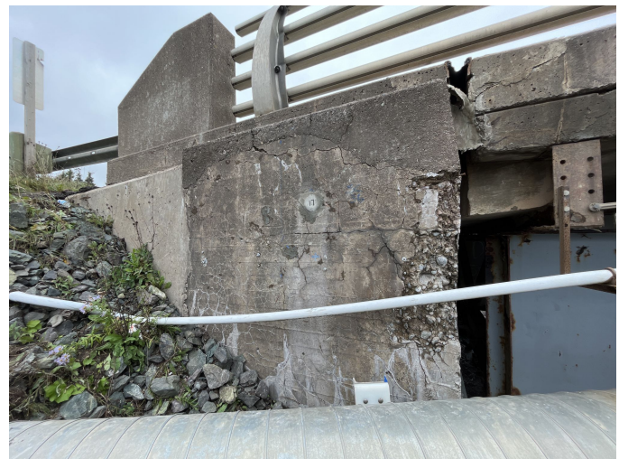
Northwest wingwall and core 17 location
