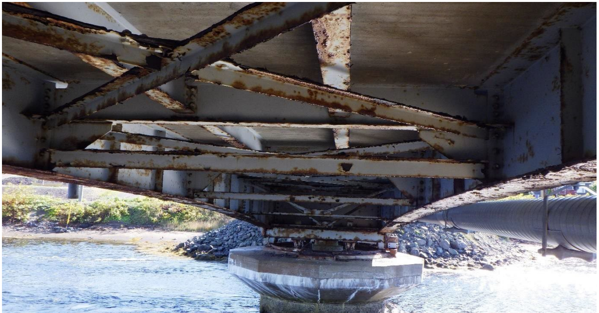
Figure 10. From Pier 3 looking at swing pier
