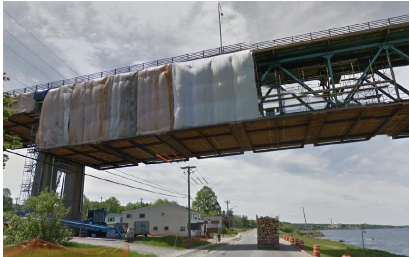
Figure 8-1: Typical Hoarding System on Mirimichi Bridge, NB (circa 2013)
