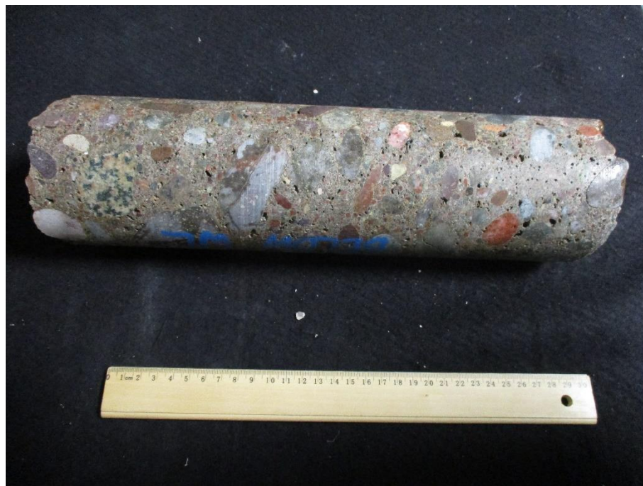
Core 29 Sampled from Pier 1 - Below high-water line in tidal zone
