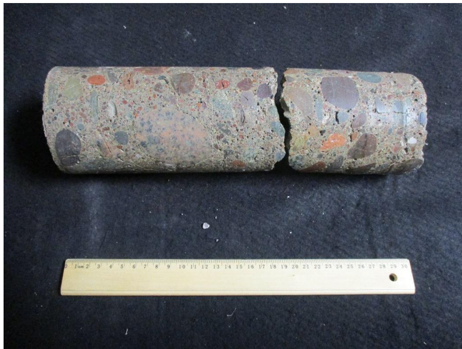
Core 12 Sampled from South Abutment – Beam Seat
