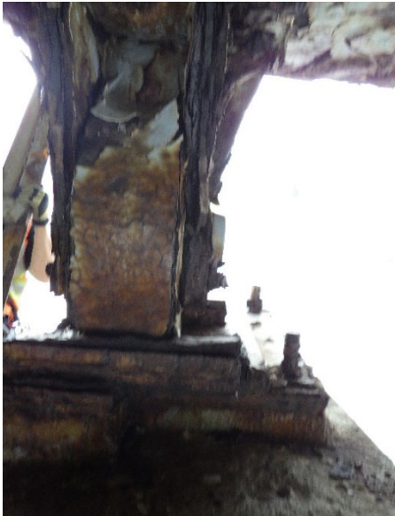
Fig #16 – Swing pier rollers.
