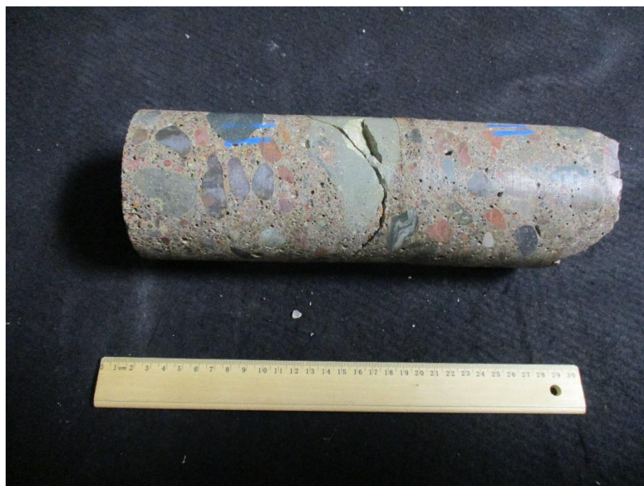
Core 11 Sampled from South Abutment – East Wing Wall
