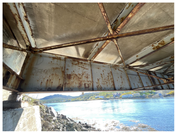
East girder looking east
