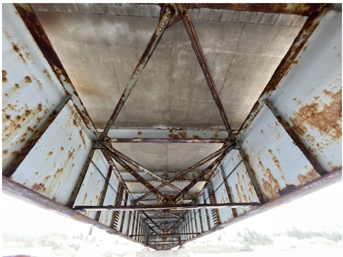
Deck soffit looking South at pier 1 in front of North abutment.
