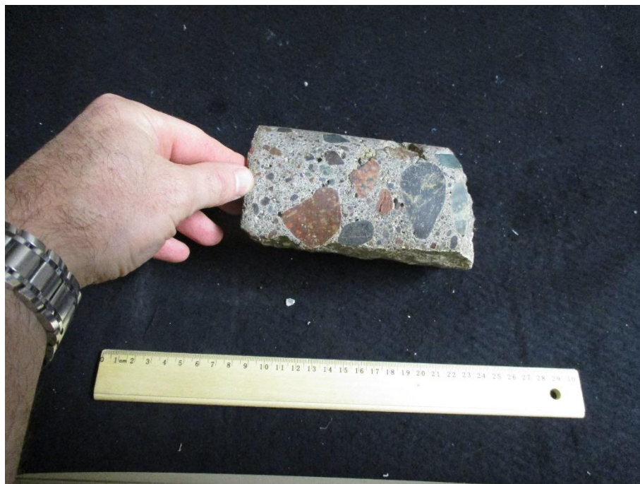
Core 33 Sampled from Swing Pier – Vertical face
