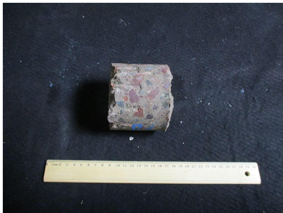
Core D2 Sampled from Bridge Deck
