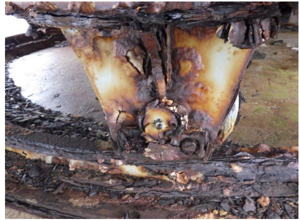
Fig #21 – Swing Pier pivot structure.
