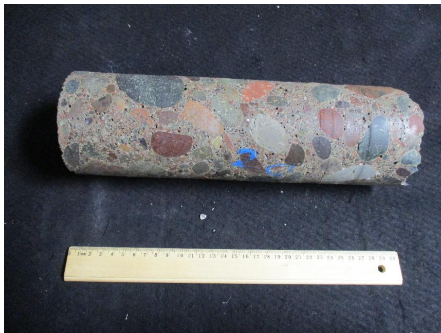
Core 20 Sampled from North Abutment - West half of foundation
