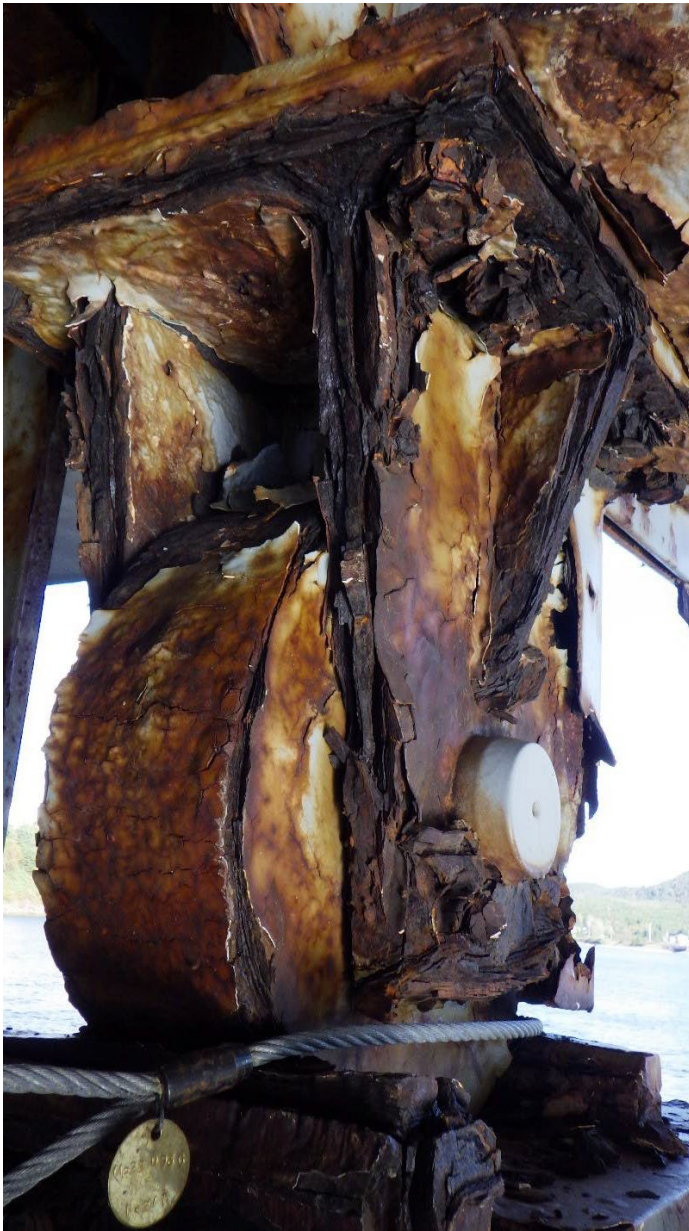
Figure 3. Bearing at swing pier
