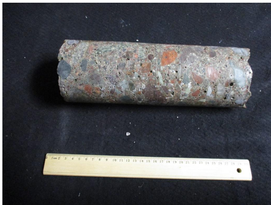
Core 25 Sampled from Pier 3 – Below high-water line in tidal zone
