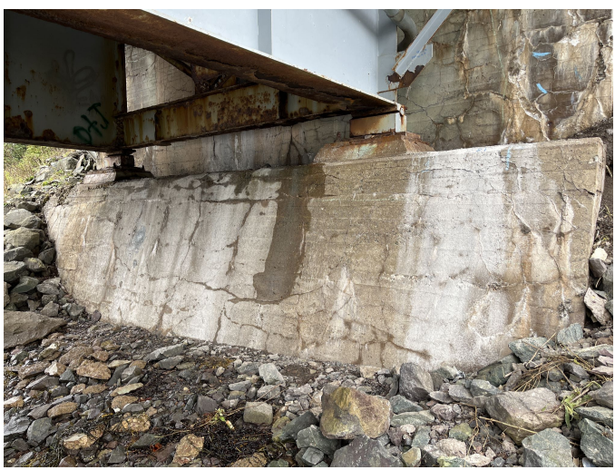
North abutment wall, core 20 location.
