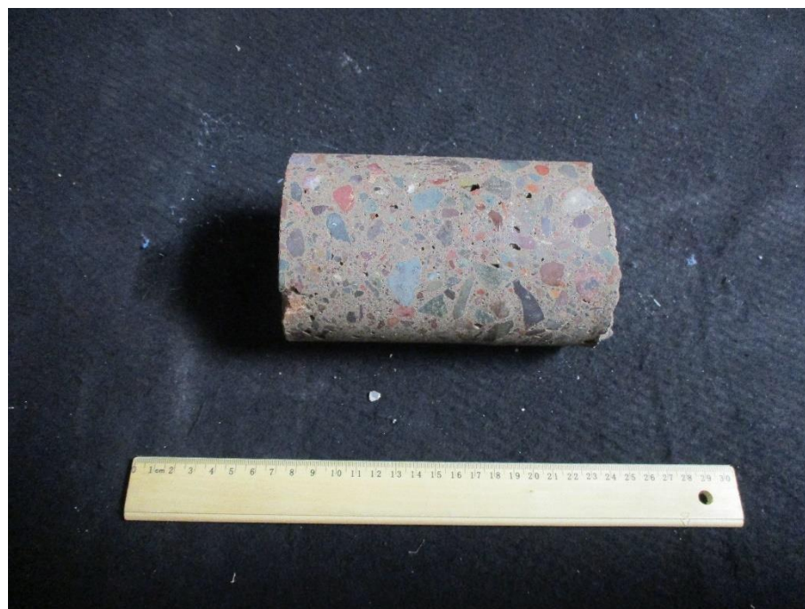
Core D5 Sampled from Bridge Deck
