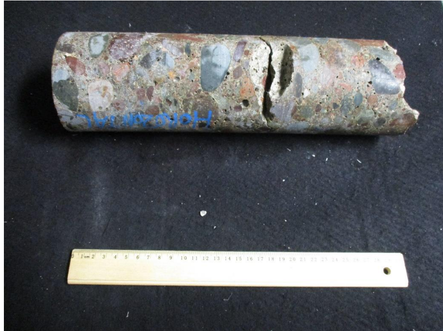
Core 28 Sampled from Pier 1 – Above high-water line
