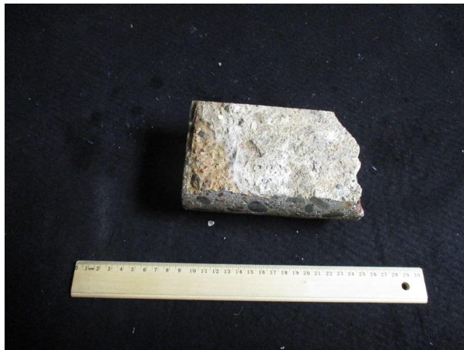
Core 33 Sampled from Swing Pier – Vertical face
