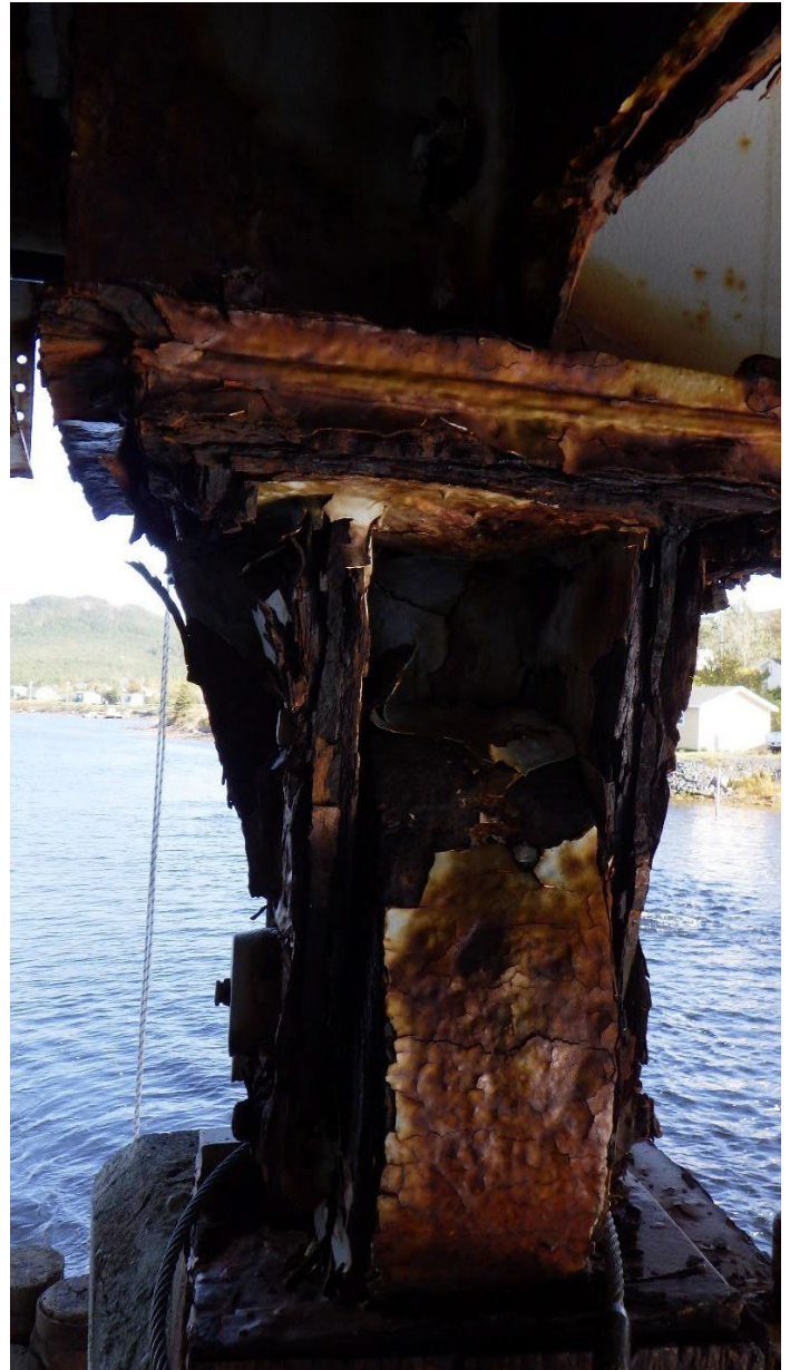
Figure 4. Bearing at swing pier
