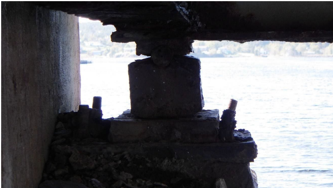
Figure 7. North side of pier three
