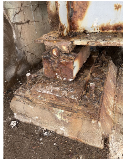
Northwest bearing looking East.
