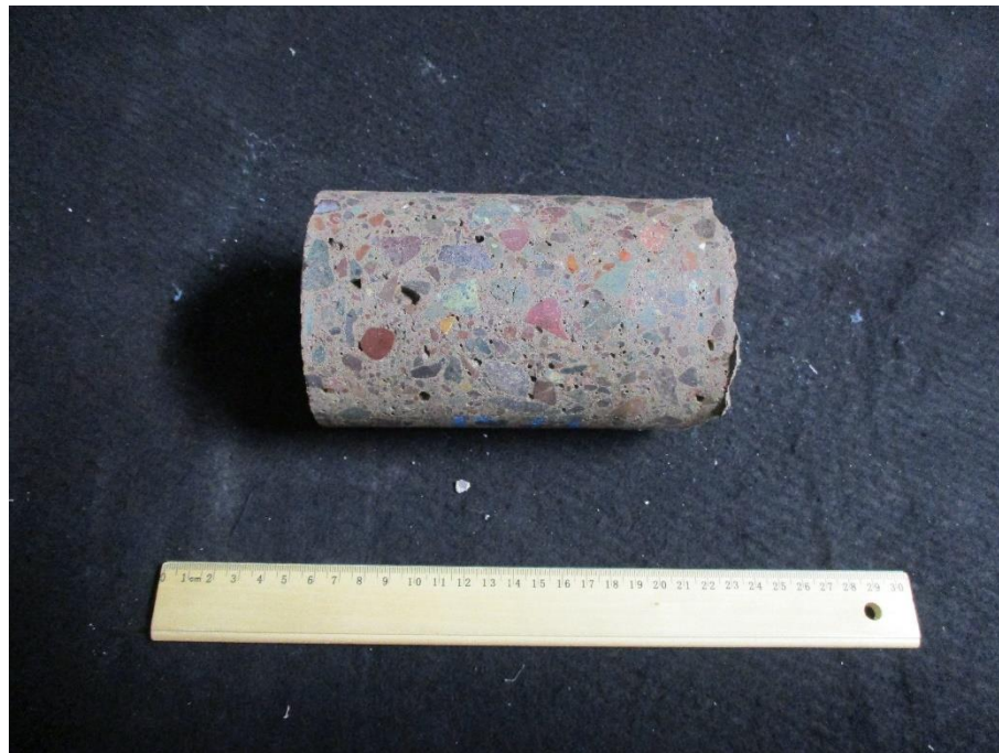
Core D4 Sampled from Bridge Deck
