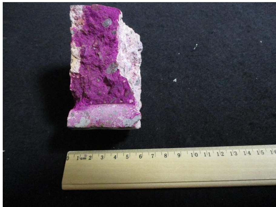
Core D8 – Carbonation Depth Sampled from Bridge Deck
