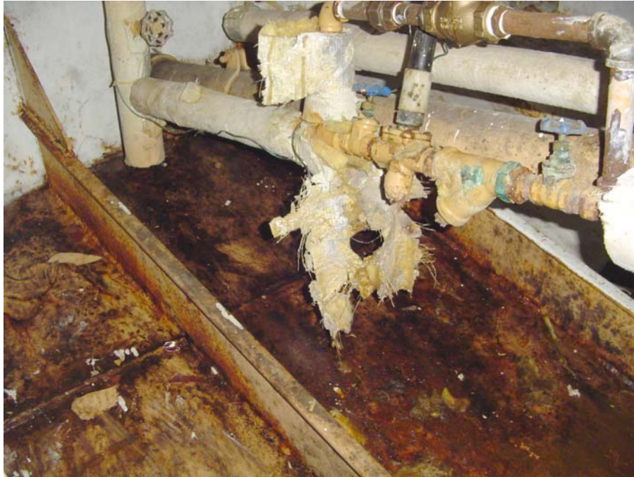
Figure 2.1: Flanders – Cofferdam Bottom Plating
