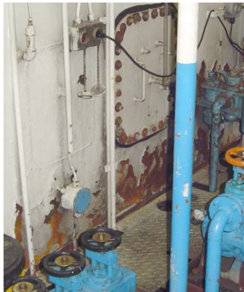
Figure 2.2: Beaumont Hamel – Fwd ER Bulkhead
