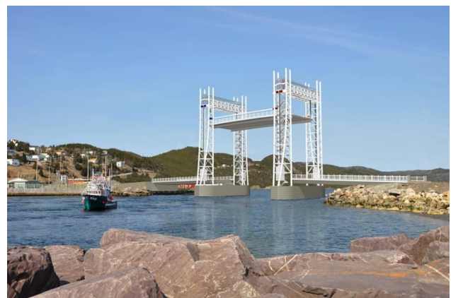
New Placentia Lift Bridge
