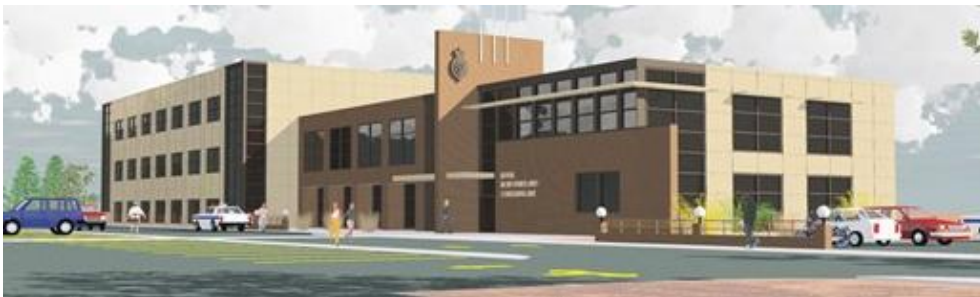
RNC Campus Redevelopment
