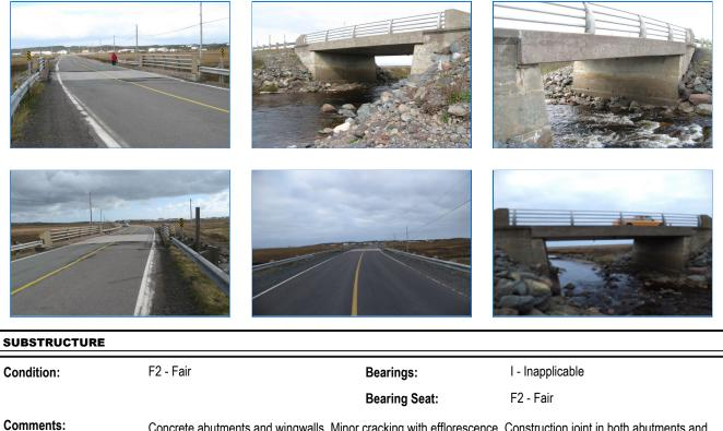
Concrete abutments and wingwalls. Minor cracking with efflorescence. Construction joint in both abutments and wingwalls is poor - some deterioration and efflorescence. Edges of bearing seats have some deterioration from
