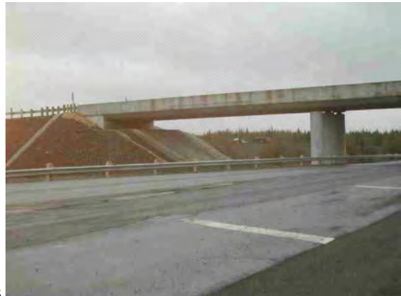
New Arnold's Cove Overpass
