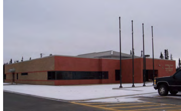
New Courthouse in Happy Valley-Goose Bay
