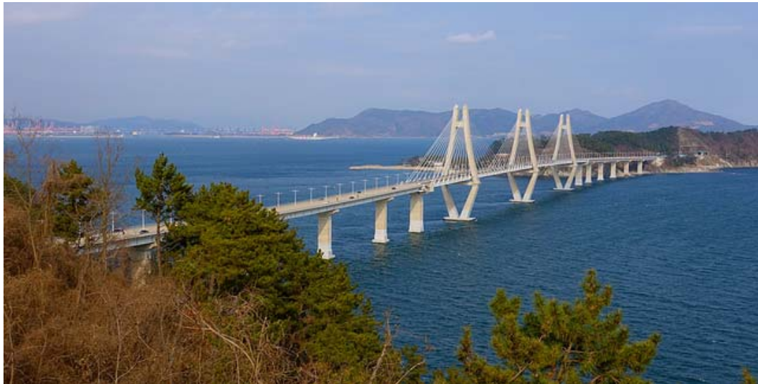
Figure 4-12: Busan-Geoje Fixed Link Bridges ( http://www.ipernity.com/doc/303473/41396014 )
