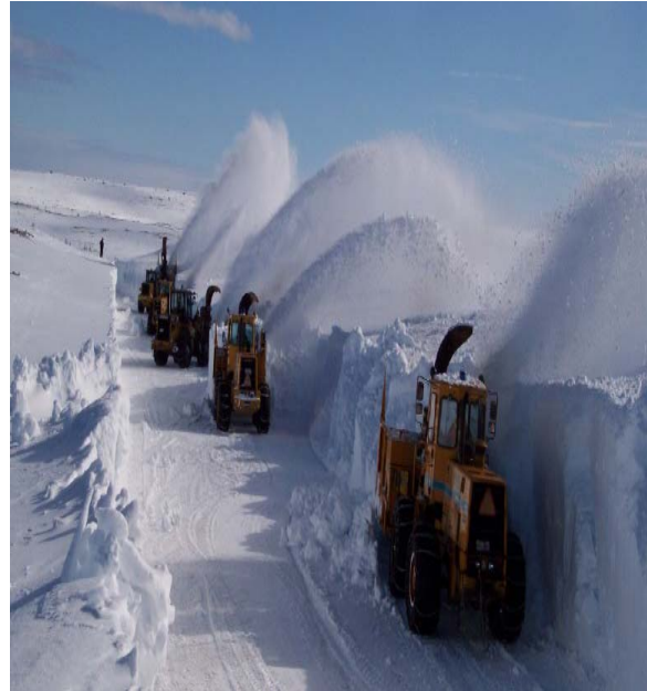
Snow blowers on Route 510 between Lodge Bay and Red Bay
