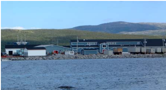
Fish Processing Facility in Makkovik
