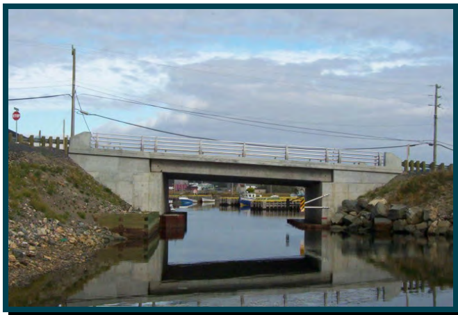
Walkham's Bridge, Bonavista
