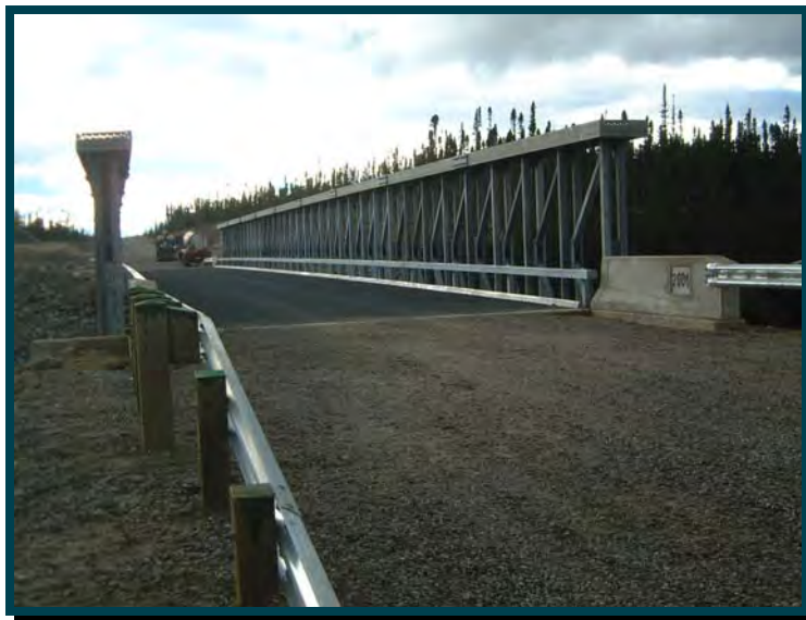
Pinware River Bridge, Labrador
