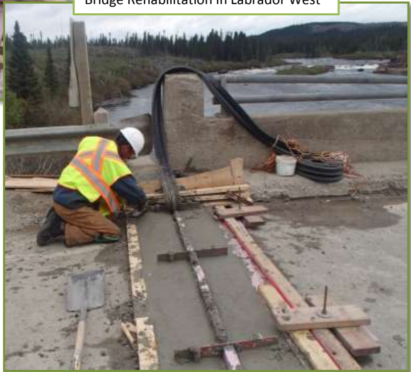
Bridge Rehabilitation in Labrador West
