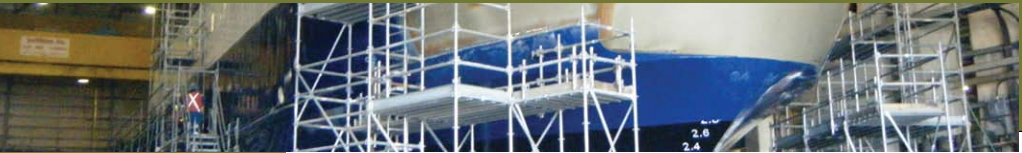
Construction of New Ferry
