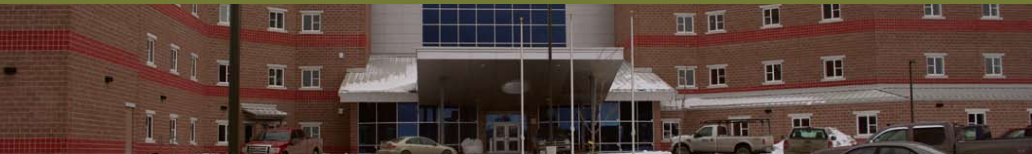
Corner Brook Long-Term Care Facility
