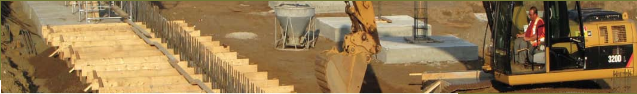
Construction of CNA - Labrador West
