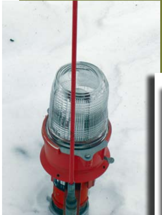
Airstrip Runway Edge Lighting
