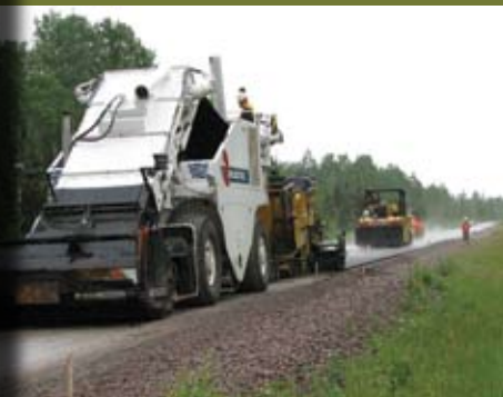
Construction of Trans Labrador Highway
